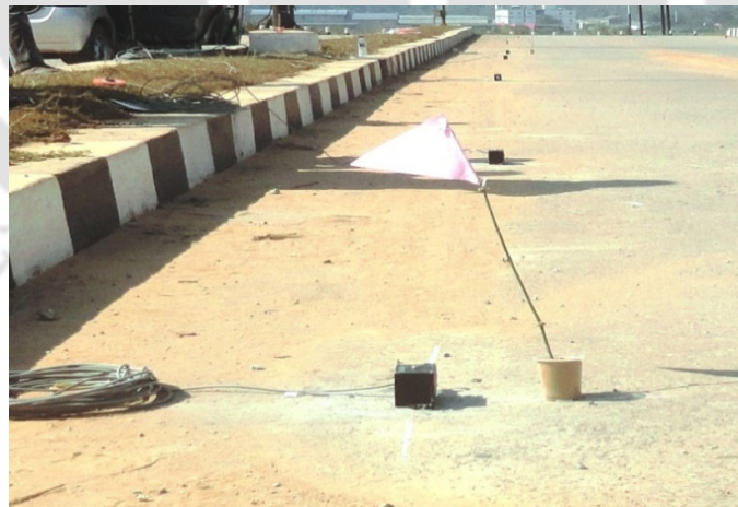
Fig. 5.10 Accelerometer glued to deck surface with data cable
