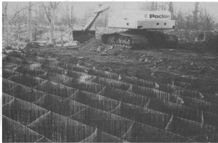
Fig. 2.12 Filling of geocell-mattress (after Bush et al. 1990)
