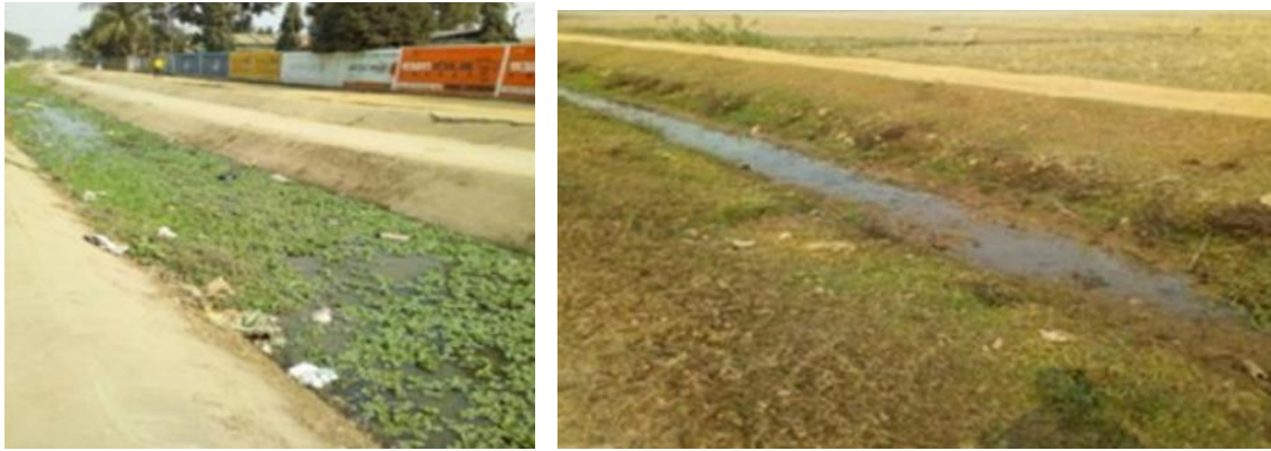
Fig. D4 Fallow lands during rabi season and dry concrete and unlined canals due to no farming activities
