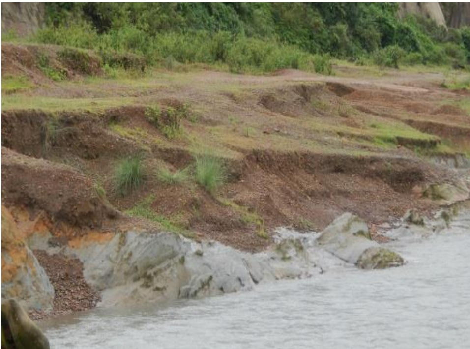
Figure 1.2 Mining site of Mathura river of Cachar district
