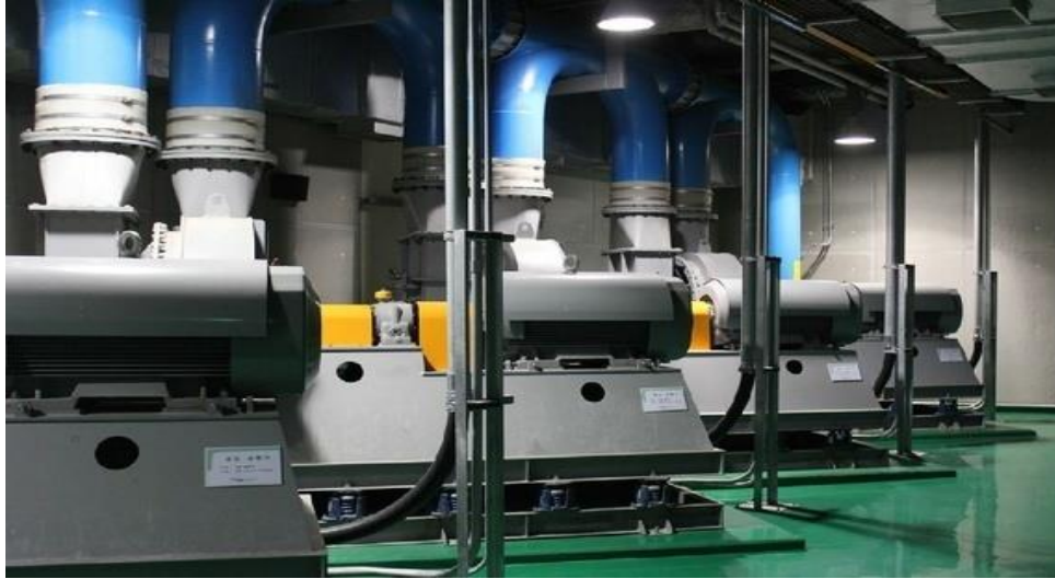
Figure 3.4 – Songdo “Third Zone Automated Waste Collection Plant,” where it is automatically processed. (Ross Arbes)
