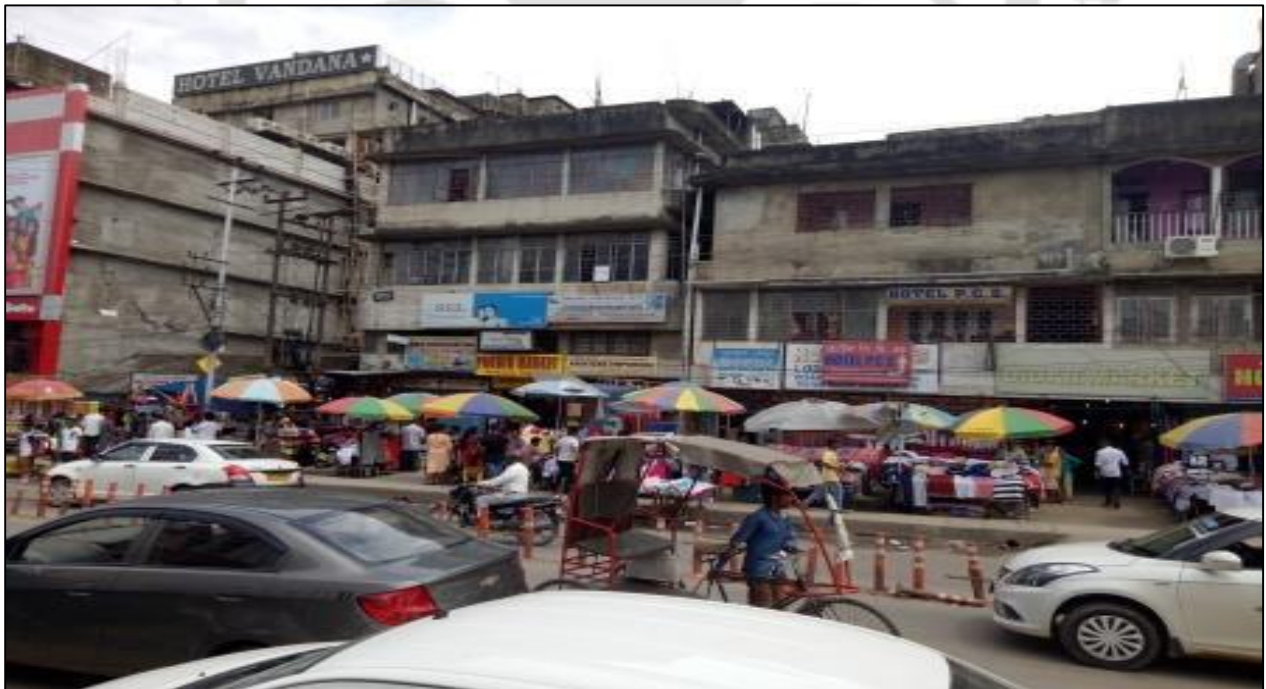
Figure 3.20 – Paltan Bazaar site photographs taken on a Tuesday @11:40 AM
