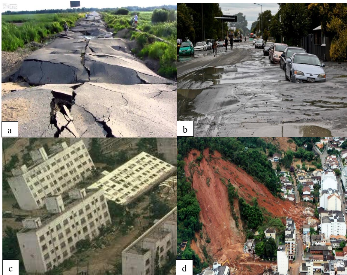
Fig. 1.1 Different modes of seismic damages (a) ground failure and (b) liquefaction during 2010 Christchurch earthquake, (c) foundation failure during 1964 Niigata earthquake (d) landslide in Brazil during 2011 disaster
