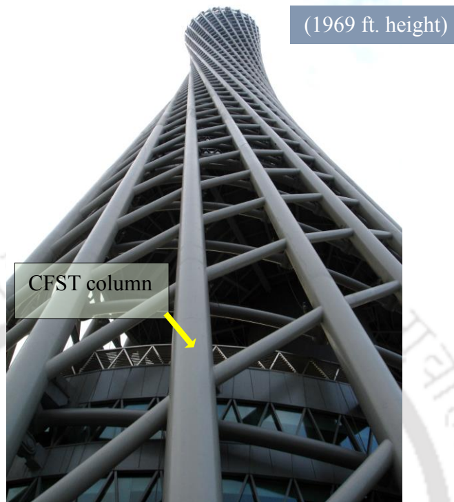
Figure 1.3: Canton Tower, China (Source: en.wikipedia.org)
