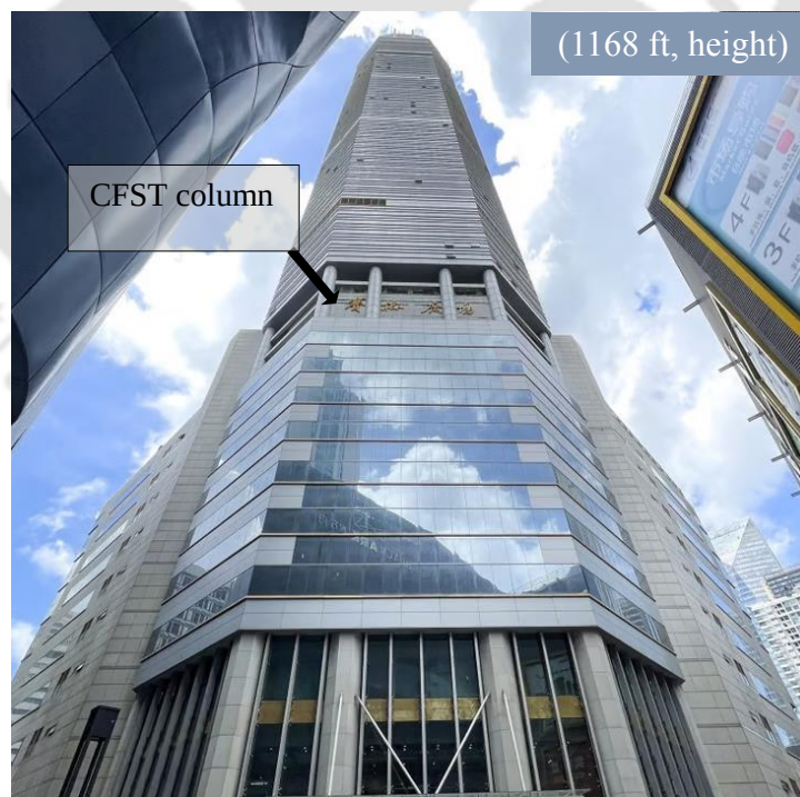
Figure 1.2: Shenzhen Plaza, China (Source: scmp.com/)
