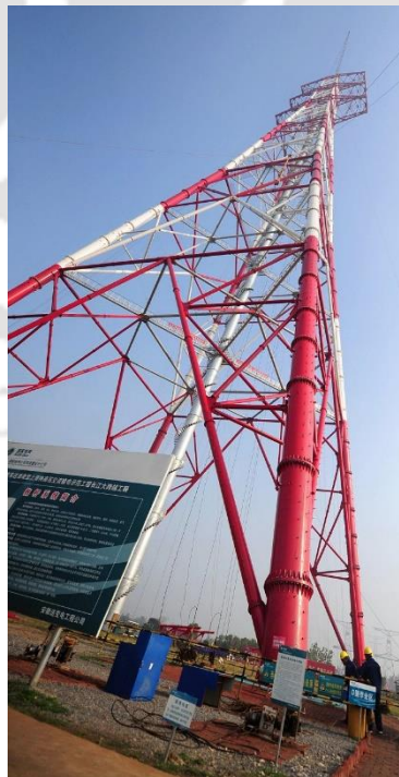
Figure 1.4: Zhoushan electricity pylon, China
