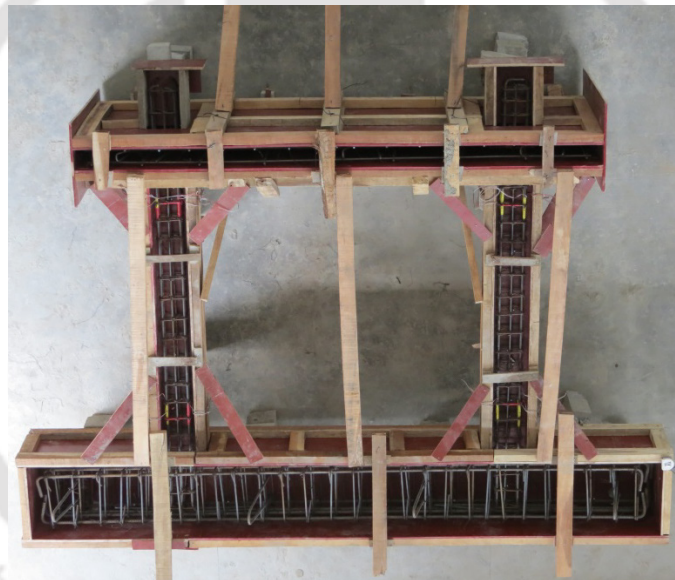
Fig. 7.5. Fabrication of formwork in the construction of RC frame.
