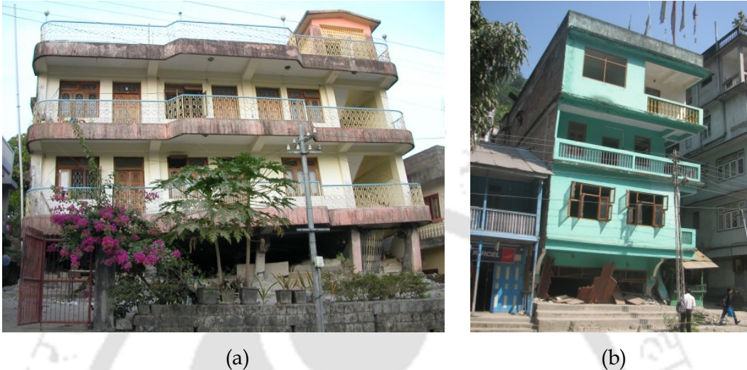
Figure 2.2 Collapse of OGS buildings during past earthquakes: (a) a three storey building in Port Blair, India after 26 December 2004 Sumatra earthquake (Kaushik and Jain 2007), and (b) a four storey building at Singtam market in Sikkim after 18 September 2011 Sikkim earthquake (Kaushik and Dasgupta 2013). Both buildings had big openings in infill walls of upper stories but still both collapsed.
