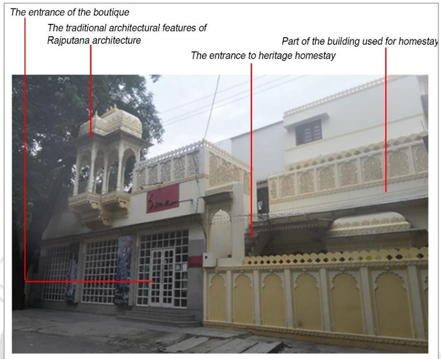
Figure 12. A haveli in Udaipur, Rajasthan, transformed into a boutique in the front for traditional clothing and a heritage homestay at the back.
