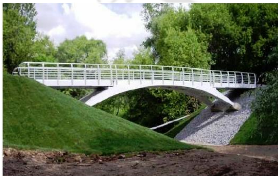
Figure 1.5: a) FRP arch footbridge; b) Railway pedestrian bridge (apatech.ru; Potyrala, 2011).
