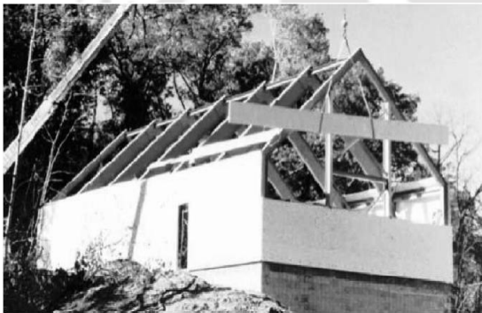
Figure 1.4: a) FRP Gable frame structure (courtesy: Strongwell; Bank, 2006); b) FRP cooling tower (Bank, 2006).
