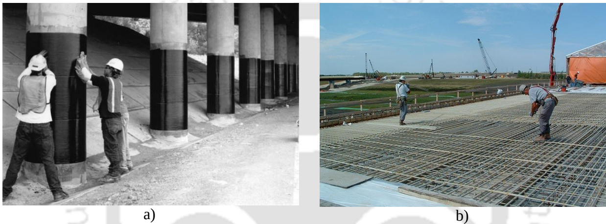
Figure 1.2: a) FRP wrapping of highway bridge columns (Bank, 2006), b) bridge deck construction using FRP reinforcing bars (owenscorning.com).
