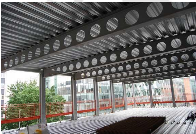
Figure 1.7: a) Cellular beams (newsteelconstruction.com); and b) Floor joist with perforation (weland.com).
