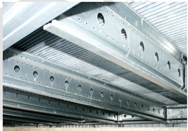
Figure 1.7: a) Cellular beams (newsteelconstruction.com); and b) Floor joist with perforation (weland.com).
