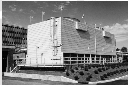
Figure 1.4: a) FRP Gable frame structure (courtesy: Strongwell; Bank, 2006); b) FRP cooling tower (Bank, 2006).
