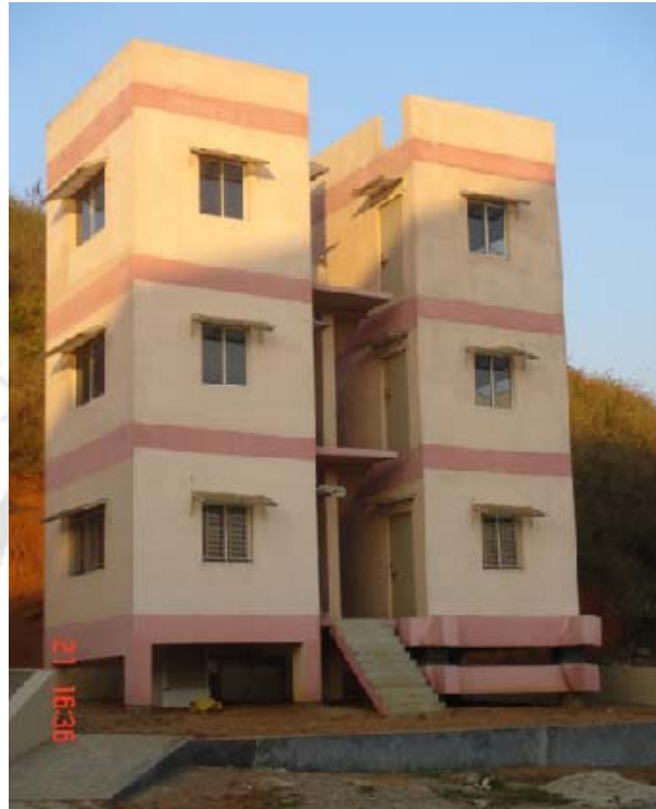
Fig. 1.10 Base isolated building at IIT Guwahati
