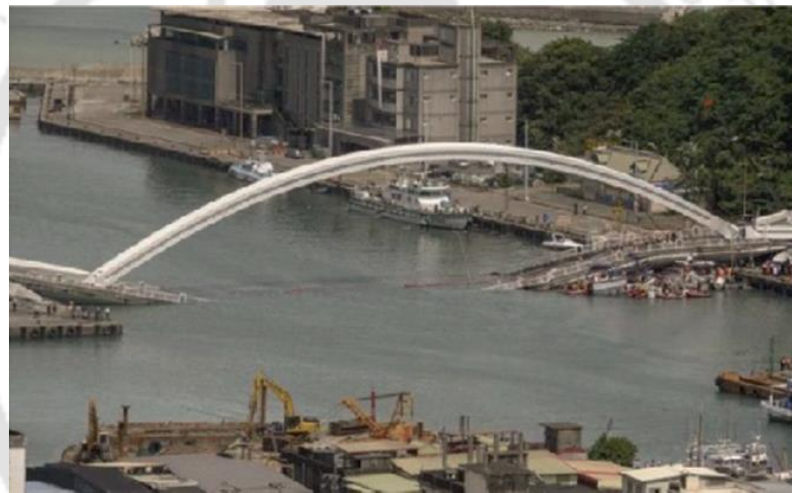
Fig. 1.2 Collapse of the Nanfang'ao bridge in Taiwan in 2019 (Source: Guowen et al., 2021)
