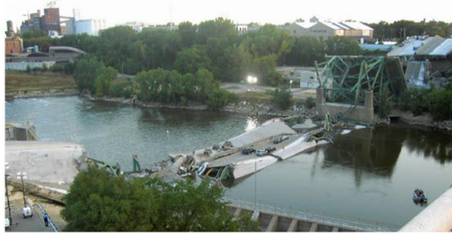
Fig. 1.1 Collapse of the I-35 W bridge in Minnesota in 2007 (Source: Deng et al., 2016)
