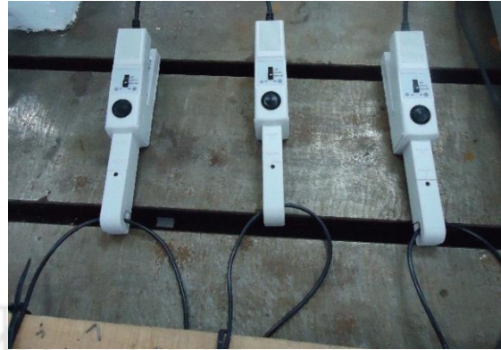
Figure 2.5: Current probes measuring motor line current
