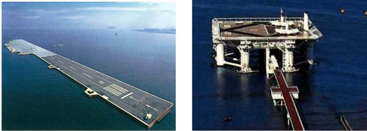
Figure 1.5: Pontoon-type VLFS and semi-submersible-type VLFS [96]
