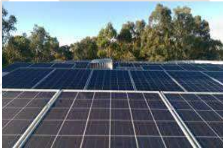
Figure 1.3: Partial shading in a real-life situation (Source: Solar Panels Melbourne Victoria, available at http://www.solarpanelsmelbournevictoria.com.au/about-us/ ).
