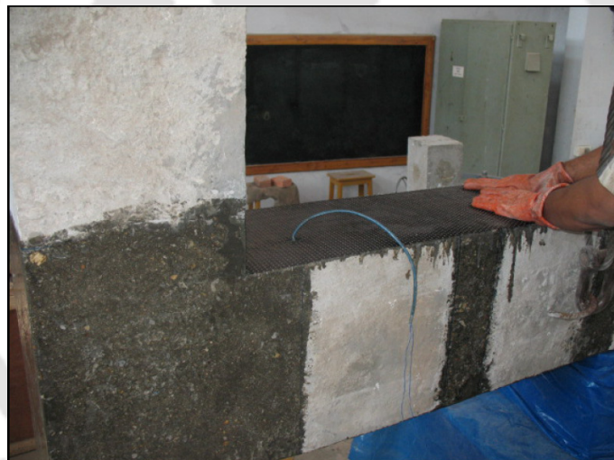
Fig. 3.11 Fixing of FRP
