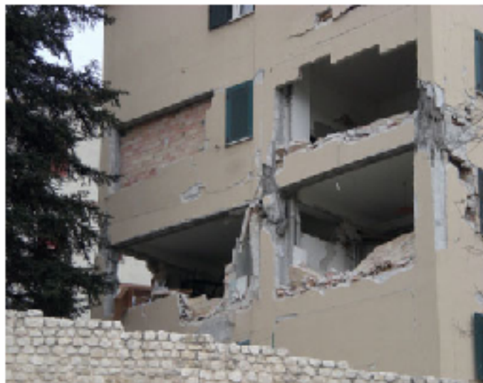
TH-951_06610408 Fig. 1.1 Beam-Column joint failure in 2009 L'Aquila Earthquake [Dr Anna Brignola, University of Genoa]
