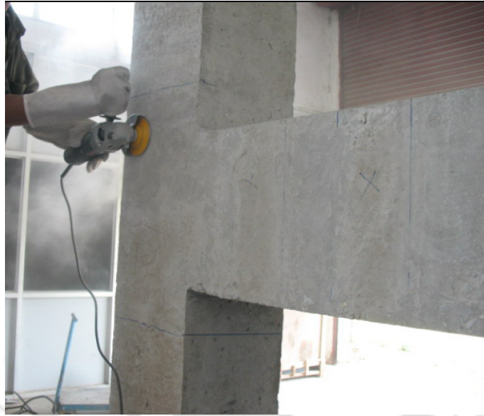
Fig. 3.10 Surface polishing by grinding machine
