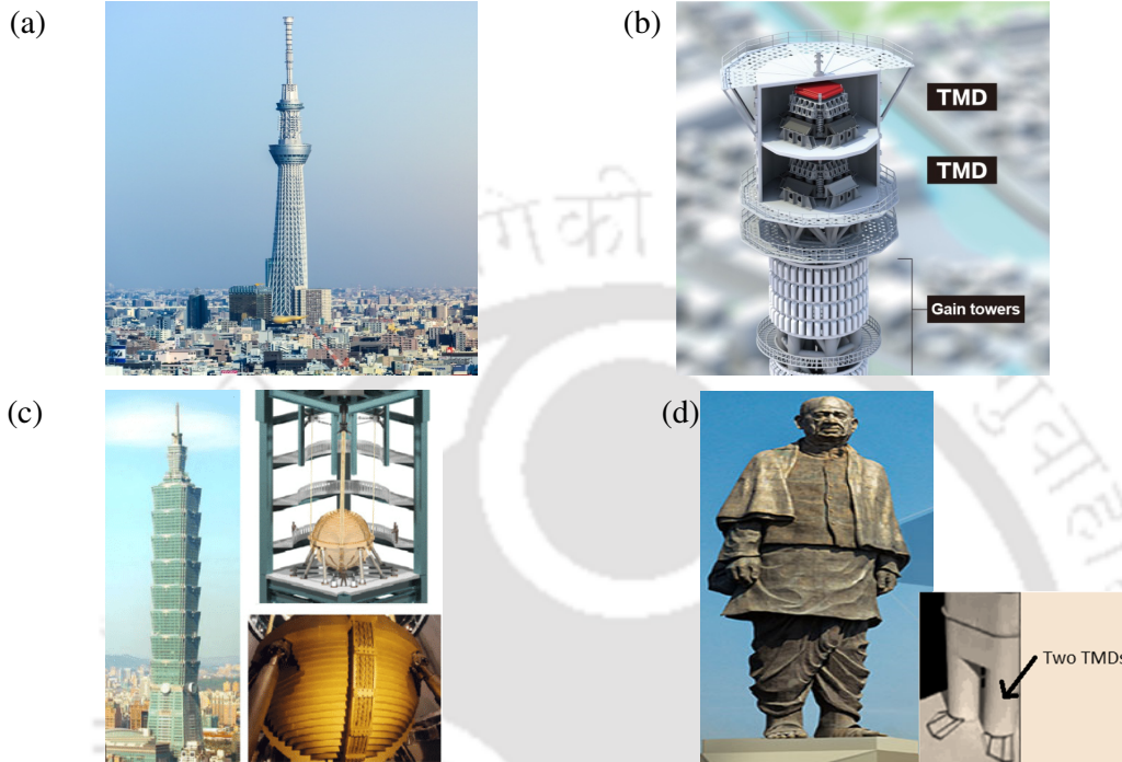
Fig. 1.8: (a) 634 m tall Tokyo sky tree, Japan (b) closed view (two TMDs) [7]. (c) Taipei 101 with a sphere-shaped TMD [48]. (d) 182 m Statue of unity in India, where two 250 tonne TMDs are used for stability against seismic and wind excitations [49].
