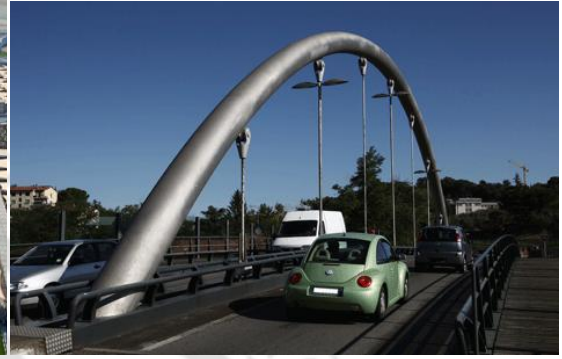
Figure 1.2: Arco Malizia bridge, Siena (Constructalia, 2017)
