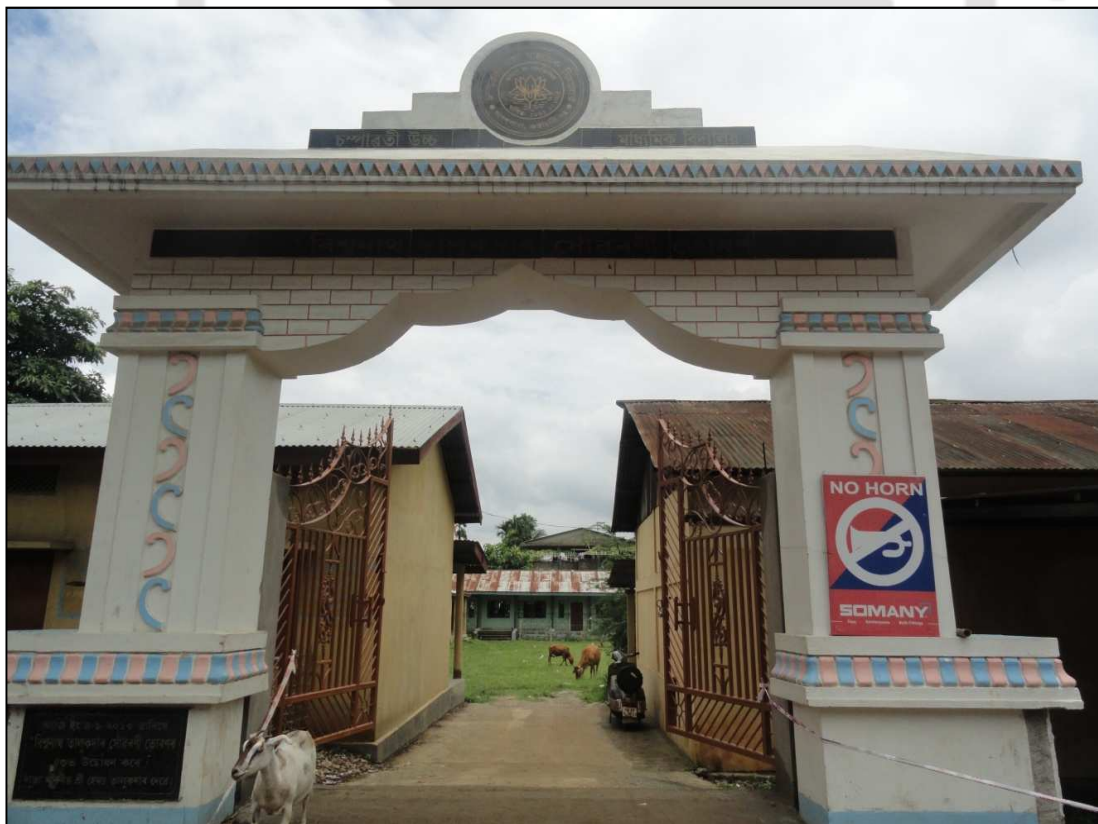
Figure 5 Main gate of Champavati Higher Secondary School.
