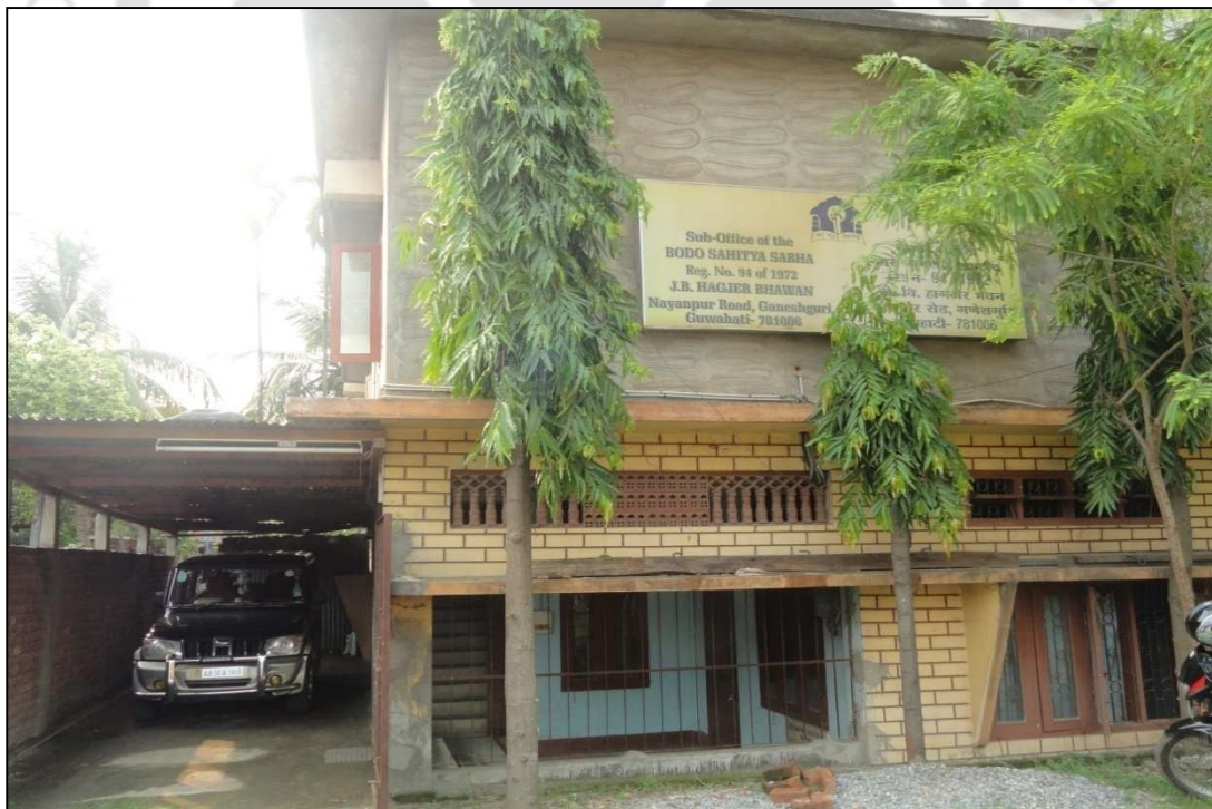
Figure 2 Office building of J. B. Hagzer Bhawan
