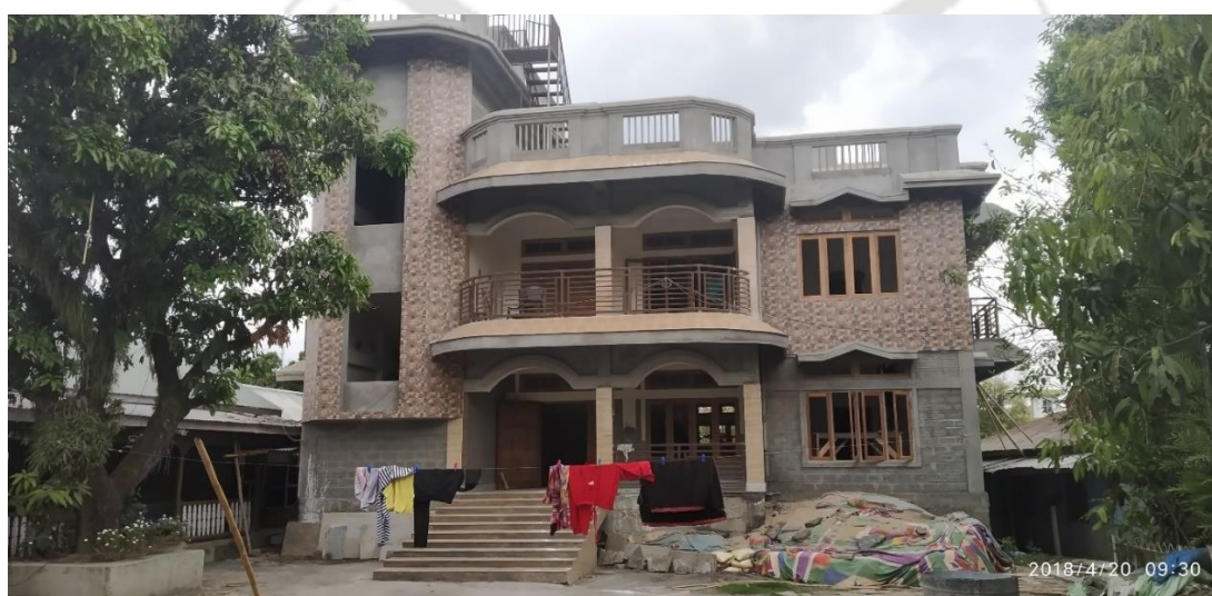
Plate 20: Pucca building in Bijang village (Photo: Author)
