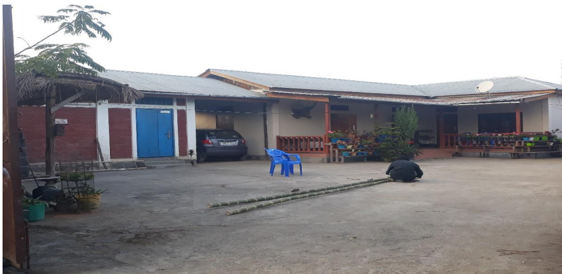
Plate 21: Tin roof with bricked wall in Bijang village (Photo: Author)
