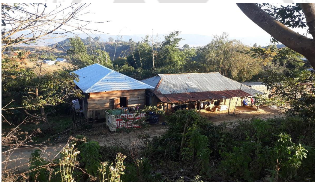
Plate 18: Tin roof with wooden wall in Teiseng village (Photo: Author)
