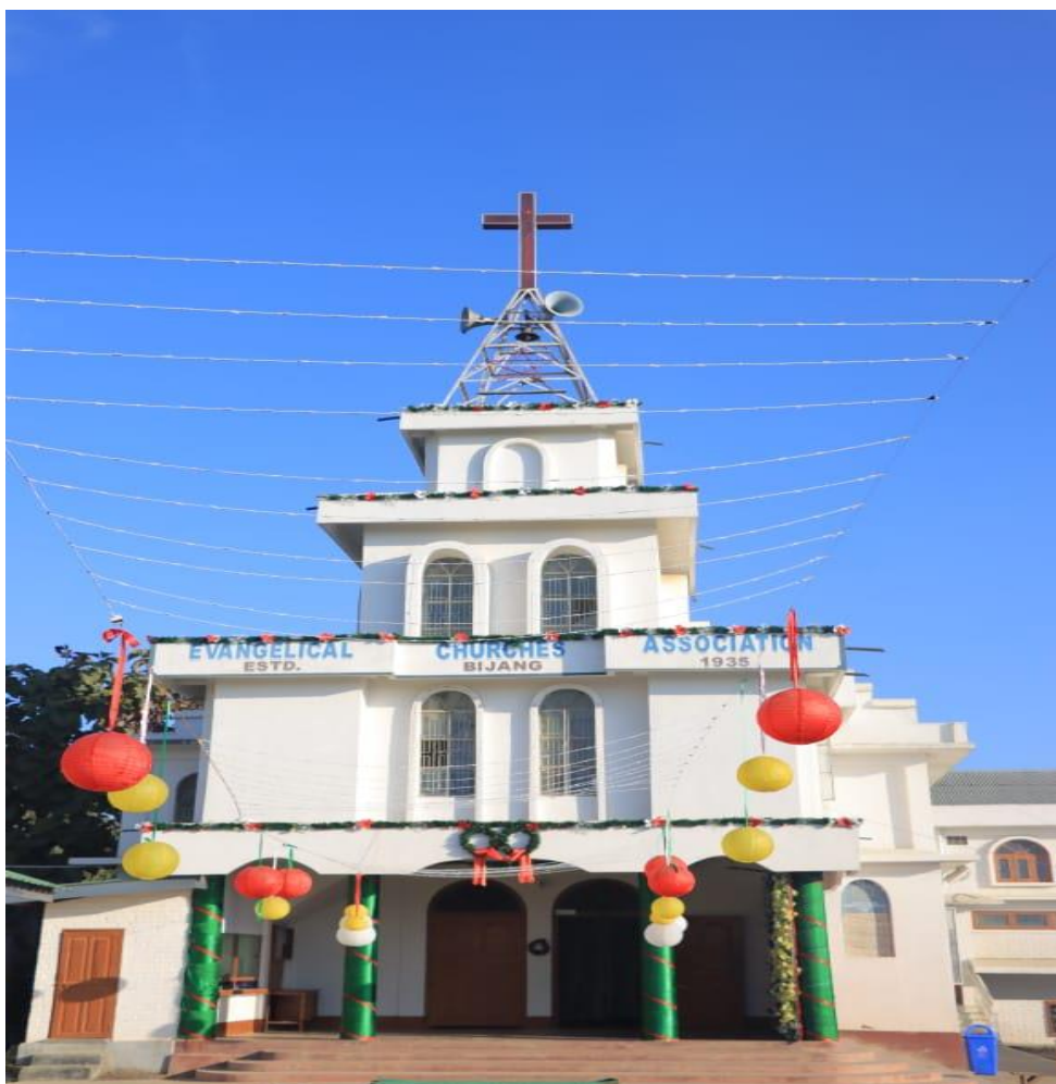
Plate 25: Church building of Evangelical Churches Association (ECA), Bijang (Photo: Author)
