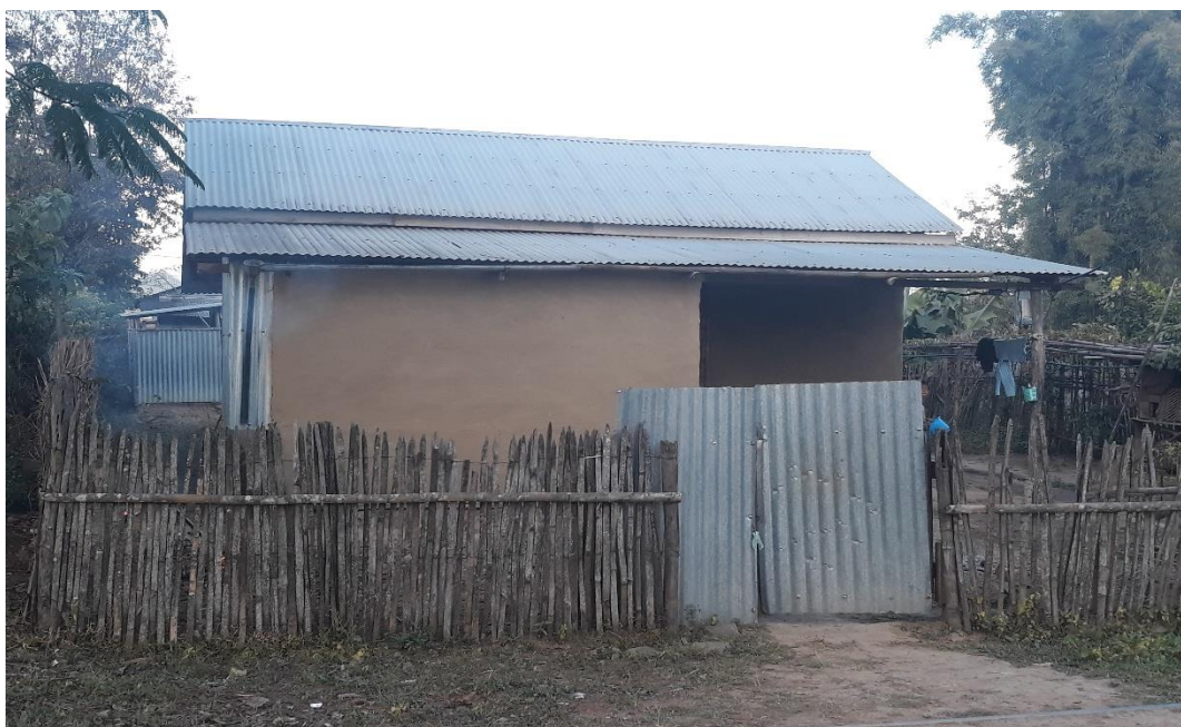
Plate 23: Tin roof with mud wall in Bijang village (Photo: Author)
