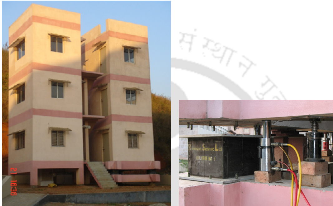
Fig. 1.10 Base isolated (HDRB) building at IIT Guwahati
