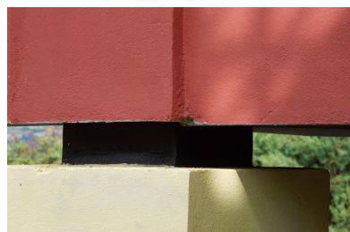
Fig. 7.1 Prototype base-isolated masonry building located at Tawang, India
