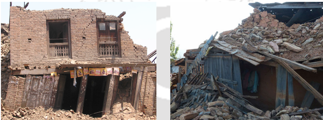
Fig. 1.11 Typical failure pattern of masonry buildings under Nepal earthquake, 2015
