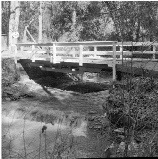
(a) Original Bridge image
