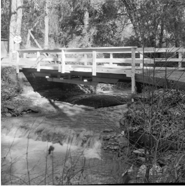
(a) Original Bridge image
