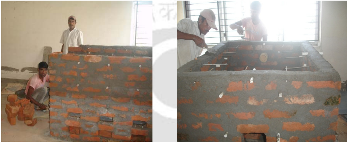
Figure 3.5: Picture of dryer constructed by local artisan
