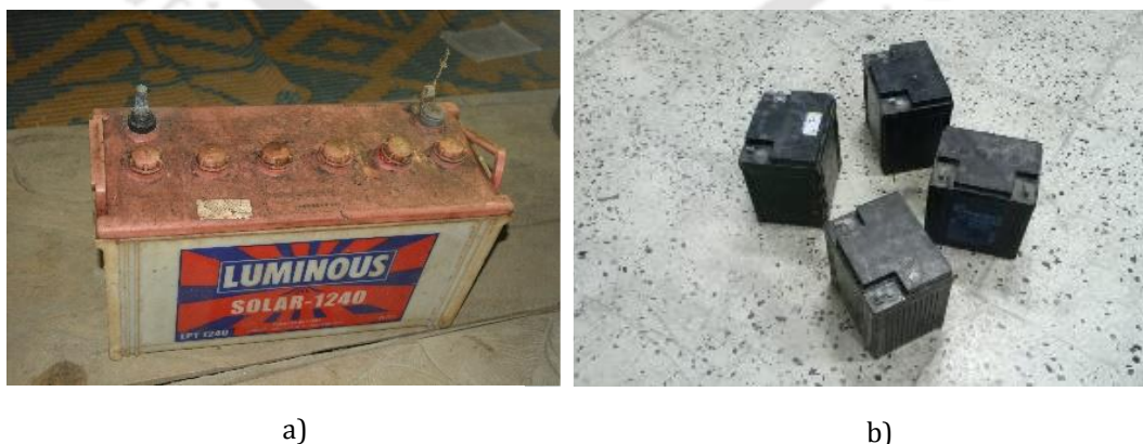
Fig 3.8. Design architecture of a) conventional system using single battery, and b) proposed discrete system using multiple small batteries of an equivalent capacity to conventional system.
