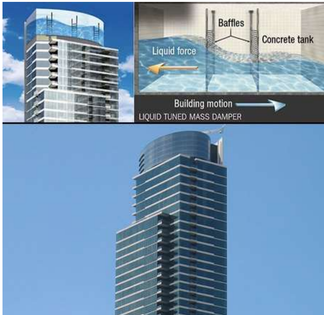
Figure 1.1. Application of TLD for mitigating dynamic response; One Rincon Hill South Tower, San Francisco. https://media.techeblog.com/images/Tuned-massdamper.jpg
