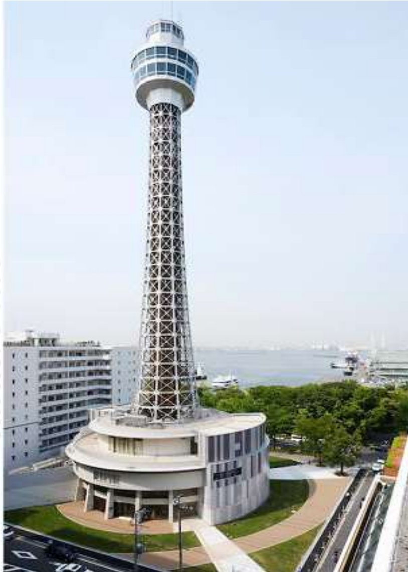
Figure 1.2. Application of TLD for mitigating dynamic response; Yokohama marine tower: Assembly of 39 multi-layered cylindrical vessels with height 0.5m and diameter 0.49m. Tamura Y et. al. (1995). https://media.Timeout.com/images/103583958/630/472/image.jpg
