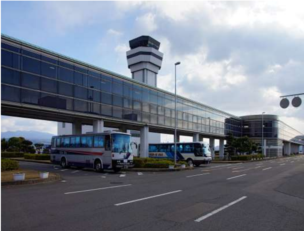
Figure 1.5. Application of TLD for mitigating dynamic response; Nagasaki airport tower: TLD consists of 25 cylindrical vessels with height of 0.5 m and diameter 0.38 m Tamura Y et. al. (1995) https://upload.wikimedia.org/wikipedia/Commons/3/38/Nagasaki_Airport_Omura_Nagasaki_pref_Jap
