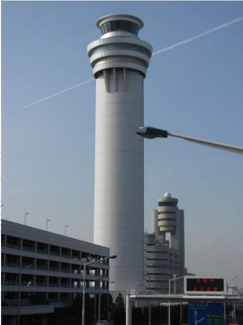
Figure 1.4. Application of TLD for mitigating dynamic response; Tokyo international airport tower. 1400 shallow cylindrical vessels of 60 cm diameter, 12.5 cm height have been installed (2001). Tamura Y et. al. (1995) https://upload.wikimedia.org/wikipedia/commons/8/8d/Tokyo_International_Airport_01.jpg
