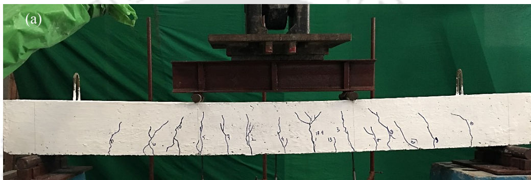
Figure 5.17 (a): Cracks in controlled beam, B2.
