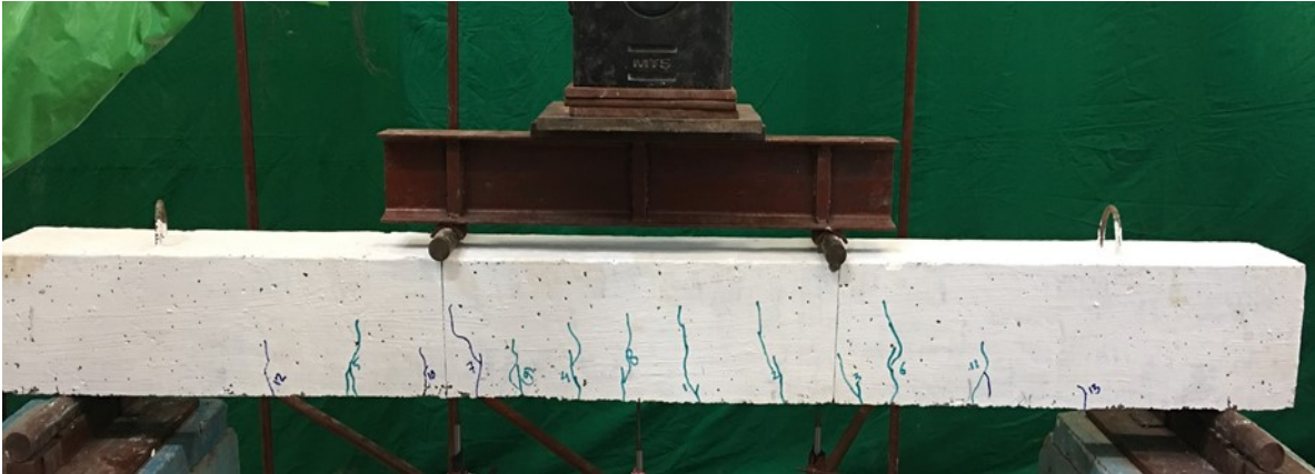
Figure 6.15 (a): Cracks in partially damaged RC beam, B13.
