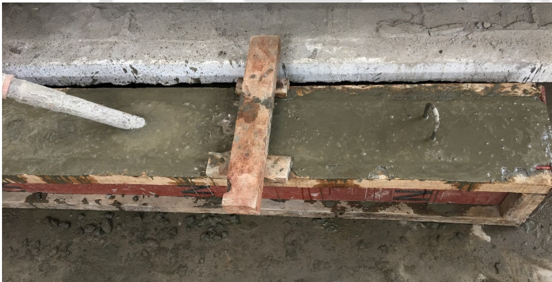
Figure 5.5: Needle vibrator used for compaction of concrete in RC beams.
