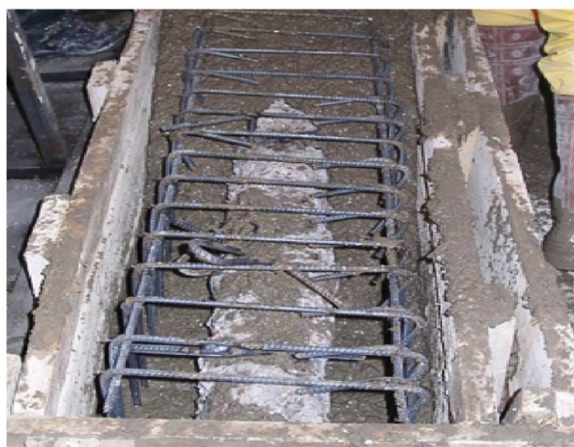
Figure 1.27: Concrete of the jacketed RC beams ( Altun [59]).
