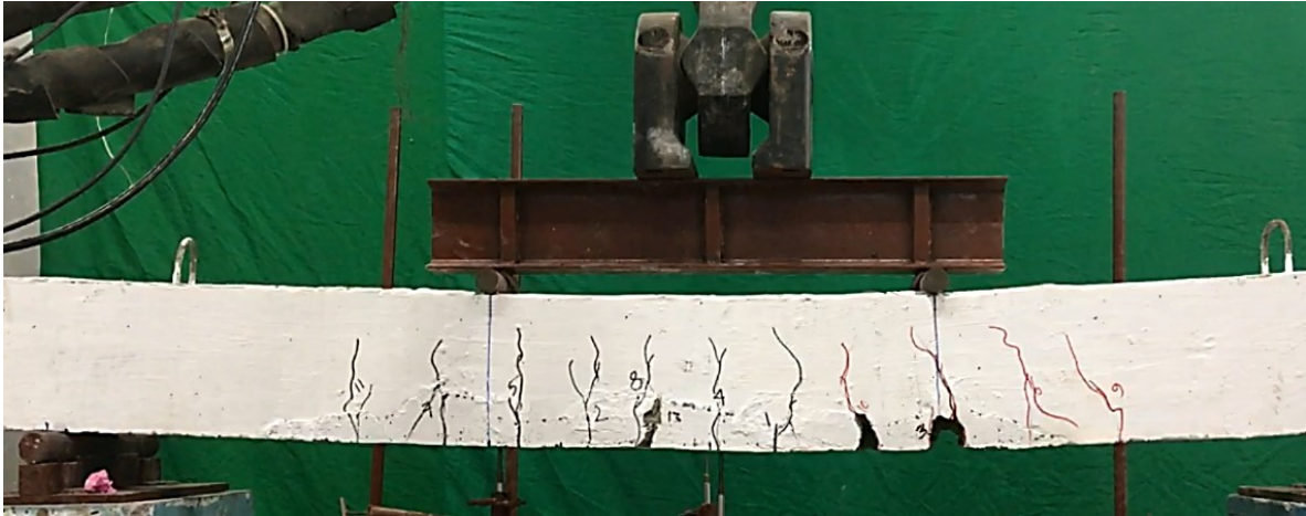
Figure 5.20: Cracks in PCM repaired beam, B6R
