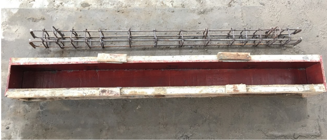
Figure 5.4: Formwork used for casting RC beams.
