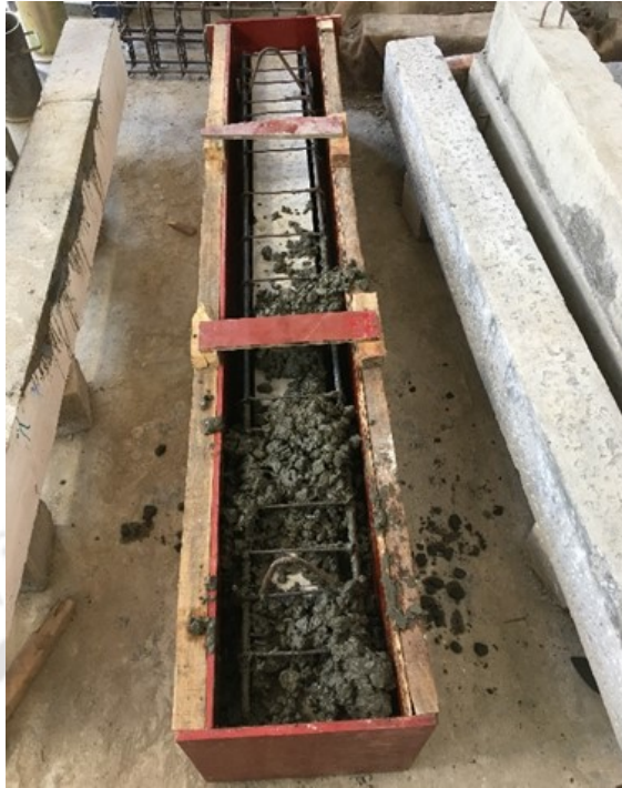
Figure 6.6: Jacketing concrete being placed inside the formwork.
