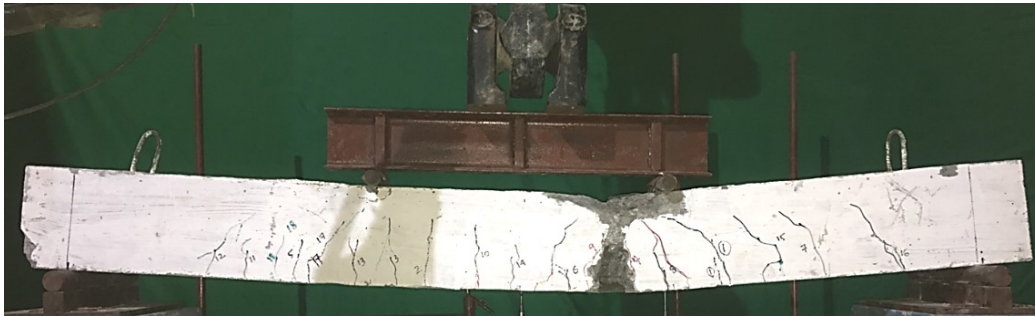
Figure 5.15 (b): Cracks in PCM repaired beam, B1R.
