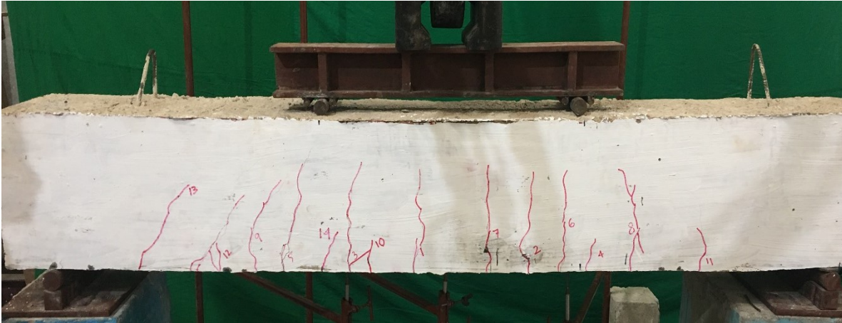
Figure 6.18: Cracks in GPC jacketed un-damaged RC beam, B16J.
