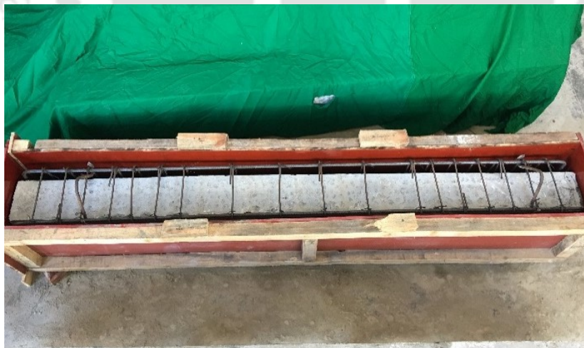
Figure 6.5: Extra reinforcement for jacketing.
