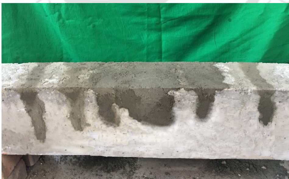
Figure 5.12: Mortar repaired damaged RC beam.
