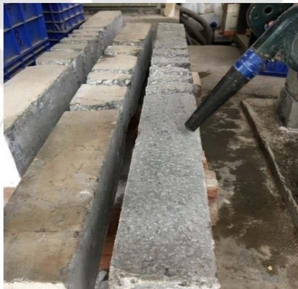
Figure 6.4 (b): Removal of dust and fine particles by air blower.
