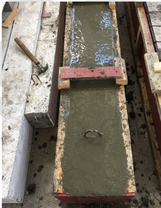
Figure 6.7: Jacketed beam ready for curing.
