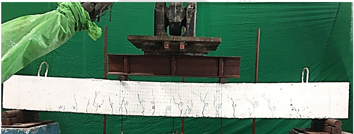
Figure 5.6: Cracks in fully damaged RC beam.
