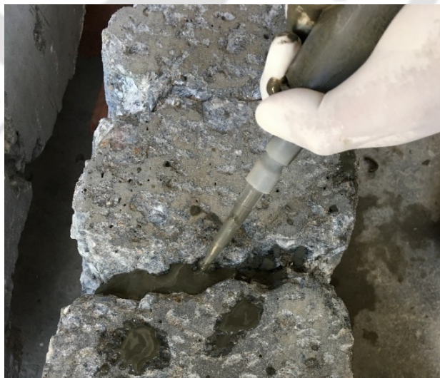
Figure 5.10: Application of repairing paste inside the cracks using syringe.
