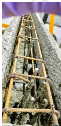
Step 8. Top beam reinforcement cage placement
