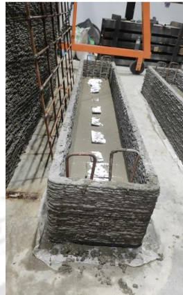
Step 2. Concrete cast up to reinforcement level
