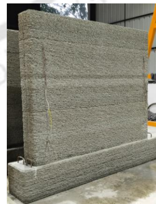
Step 11. Full wall (with strain gauges wire coming out)
