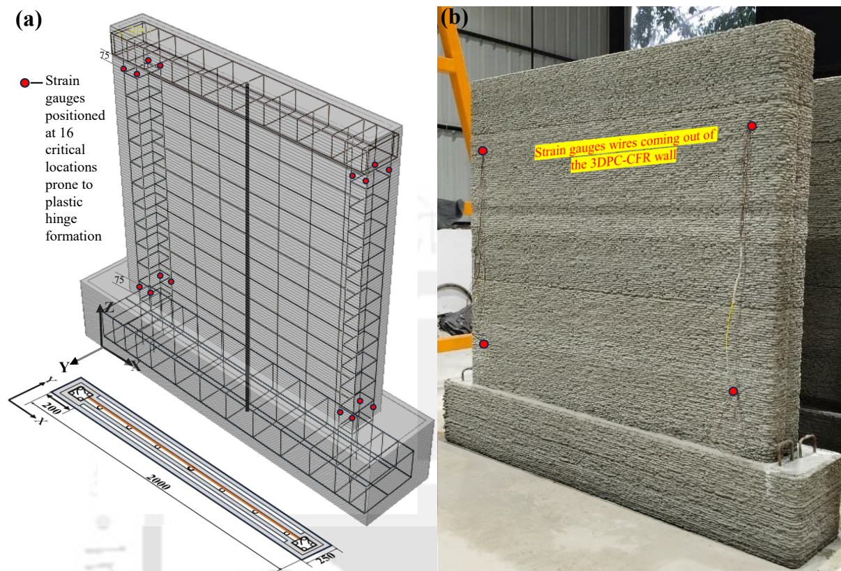
Fig. 6. 7. (a) Modular reinforcement cage showing the complete 3D configuration with strain gauges with cross-sectional infill pattern; (b) 3DPC–CFR wall with visible strain gauge wires
