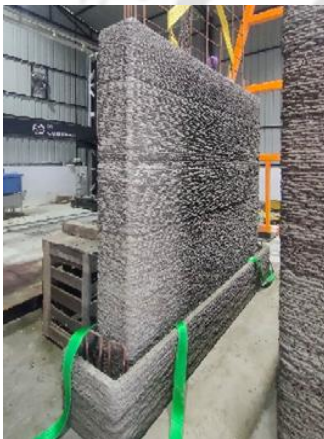
Step 5. Reinforcement cage insertion in the wall (Column reinforcement with central single layer grid reinforcement placement)
