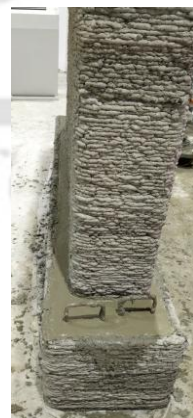
Step 10. Casting of the bottom beam
