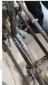
Step 6. Applying the epoxy on the surface of strain gauges
