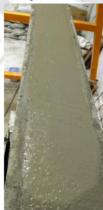
Step 9. Casting of the concrete from the top beam
