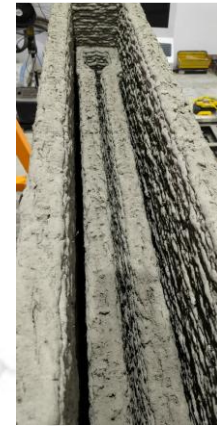
Step 4. Full wall layer printing (top view of the wall)
