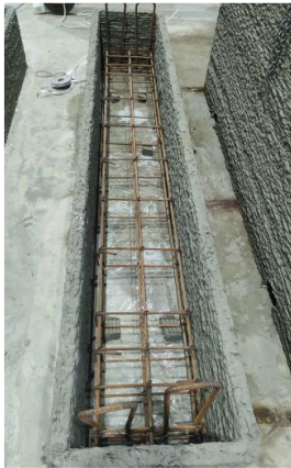
Step 1. Bottom beam mould fabrication and reinforcement cage placement
