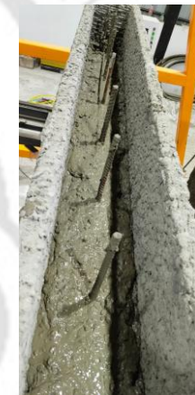
Step 7. Casting till wall level
