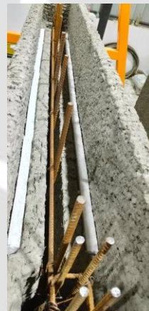
Step 5. Reinforcement cage insertion in the wall (Column reinforcement with central single layer grid reinforcement placement)
