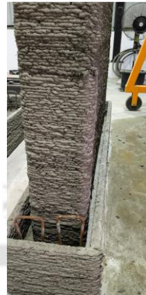
Step 3. Wall layer printing on above of the cast concrete level
