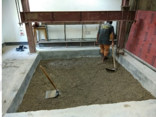
Figure 3.10: Laying of the base material
