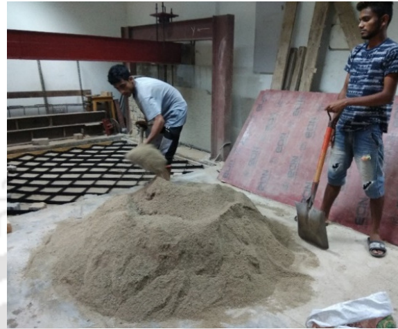
Figure 3.12: Hand mixing of bedding sand
