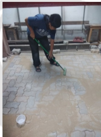
Figure 3.19: Jointing sand filling
