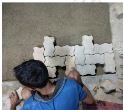
Figure 3.15: Block arrangement
