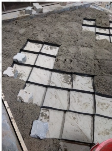
Figure 3.13: Filling in bedding sand
