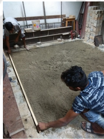
Figure 3.14: Leveling bedding layer
