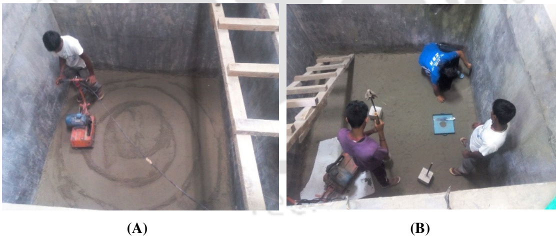
Figure 3.9: Construction of the foundation: (A) compaction (B) density check
