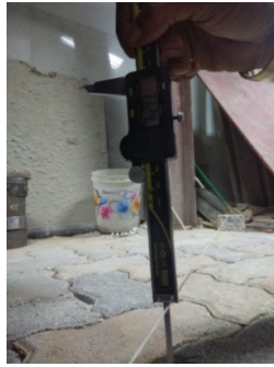
Figure 3.17: Surface Profile checking
