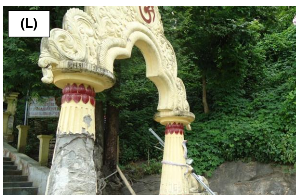
Figure 2.5 (L) Main entrance (U1) in Umananda River Island
