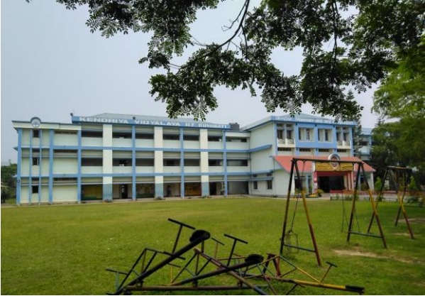
KVS School Building
