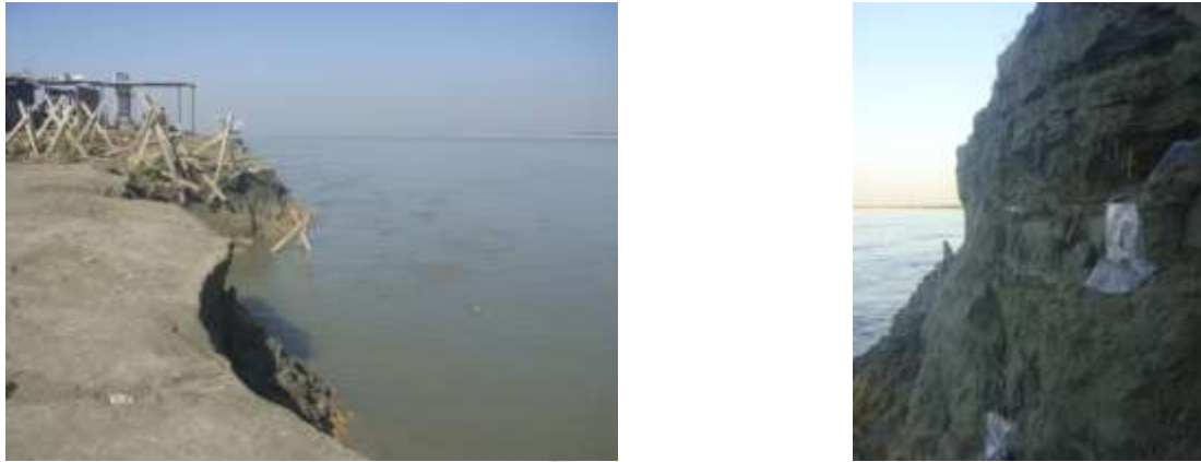
Figure 6.4 Loose structure of river bank in erosion site C
