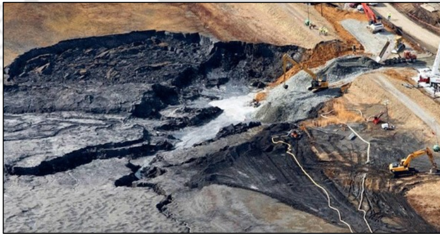
Figure 2.4 Coal Ash earthen dam breach on River Dan, North Carolina, 2014 ( http://duluthreader.com/articles/2018/04/26/13157_a_sampling_of_16_earthen_dam_failures )
