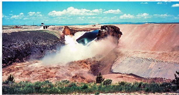
Figure 2.7 Historic Teton dam failure in 1976, Idaho, USA ( https://history.info/on-this-day/1976-collapse-of-the-teton-dam-in-idaho/ )
