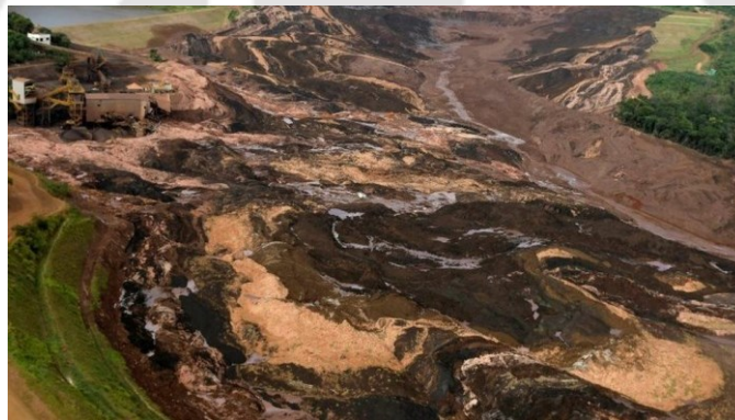
Figure 2.6 Brumadinho dam disaster, Brazil, 2019 ( https://www.bbc.co.uk/news/resources/ids-sh/brazil_dam_disaster )
