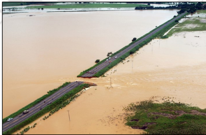
Figure 2.2 Failure of Campos's dos Goytacazes dam, Rio de Janeiro, Brazil, 2012
