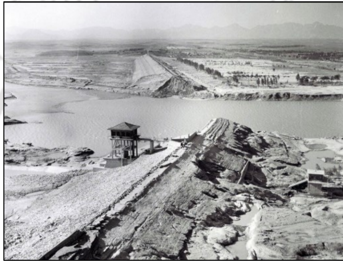
Figure 2.1 Failure of Banqiao Reservoir Dam, Henan, China, 1975
