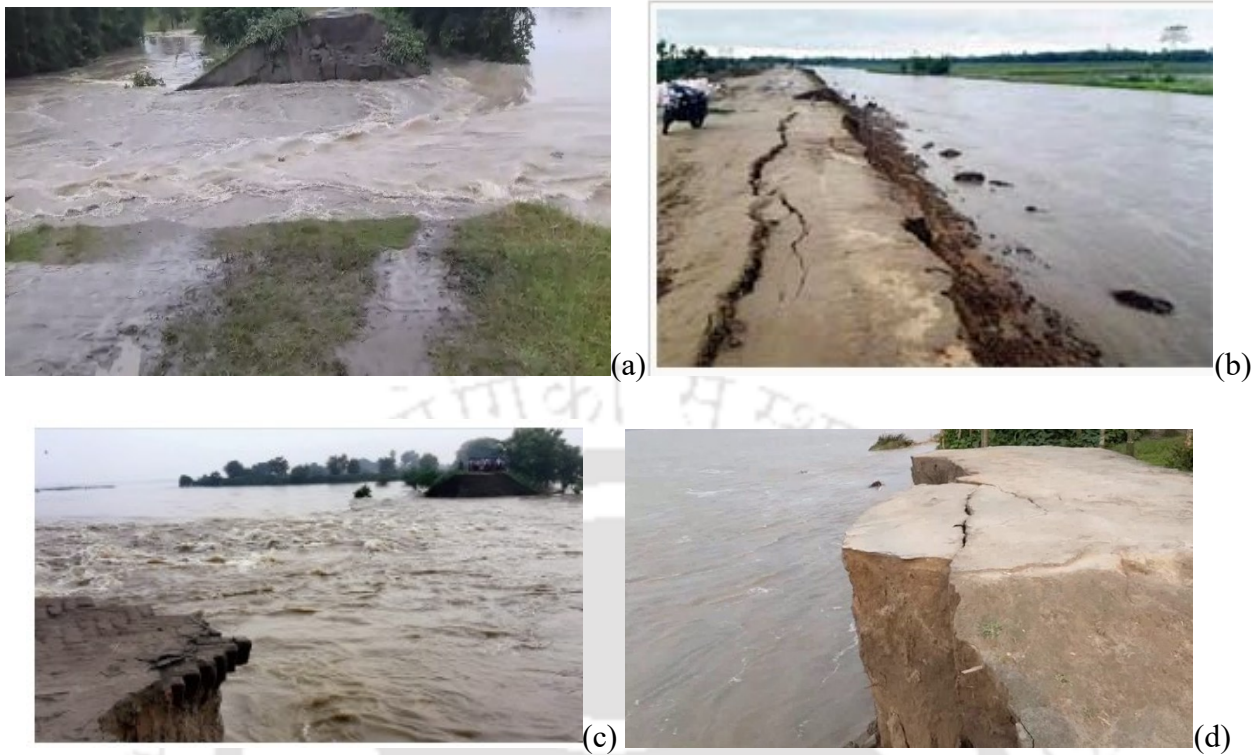
Figure 1.1 A glimpse to some of the failures of earthen embankment dams in Assam, India, 2019
