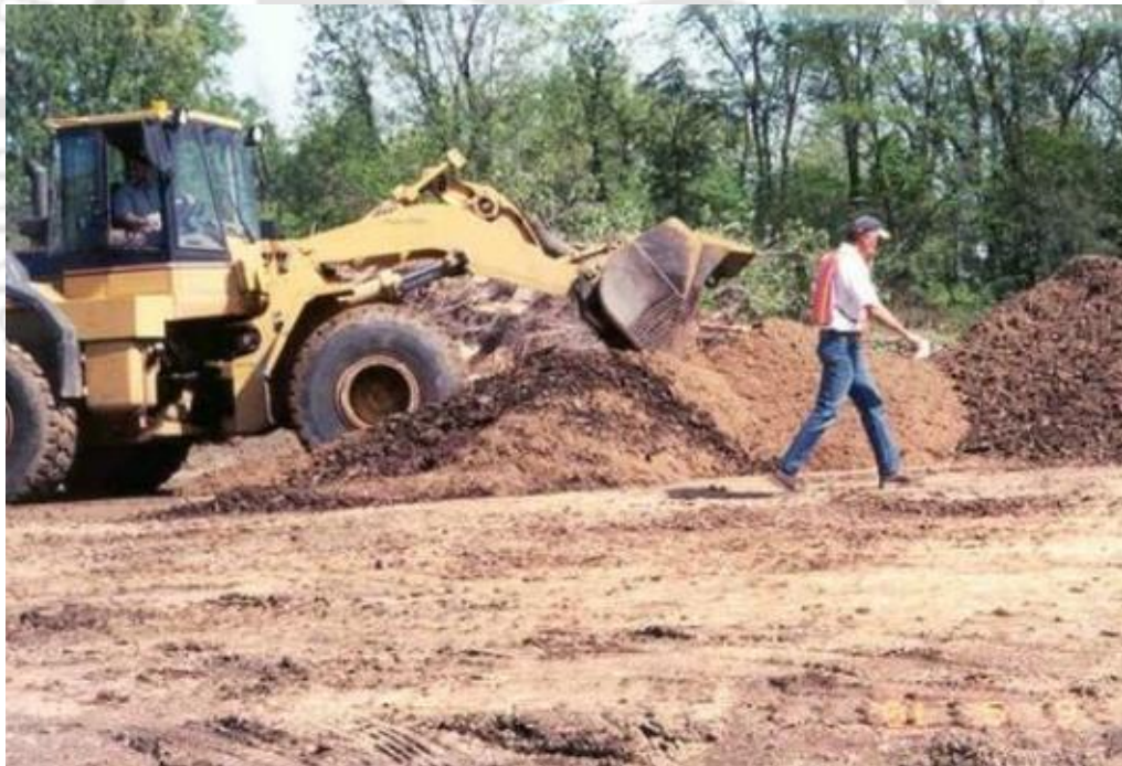
Fig. 2.24 Sand - tire chip mixture (75/25) (after Yoon et al. 2006)
