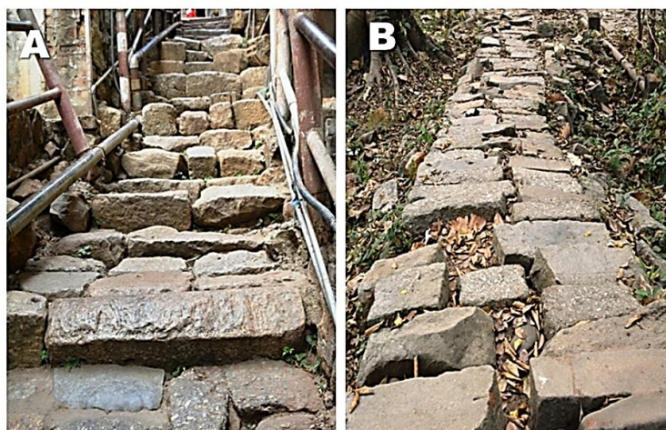
Figure 24. Example of undressed stone fragments in the archaeological site of Kamakhya temple: Figure A) & B) Undressed stone blocks in the stairways located on the backside of the main Kamakhya temple and in the western pathway.
