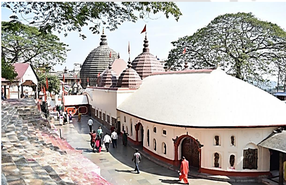
Figure 2. The Kamakhya temple, representing the unique Nilachala style of Hindu temple architecture known for its bulbous polygonal dome.
