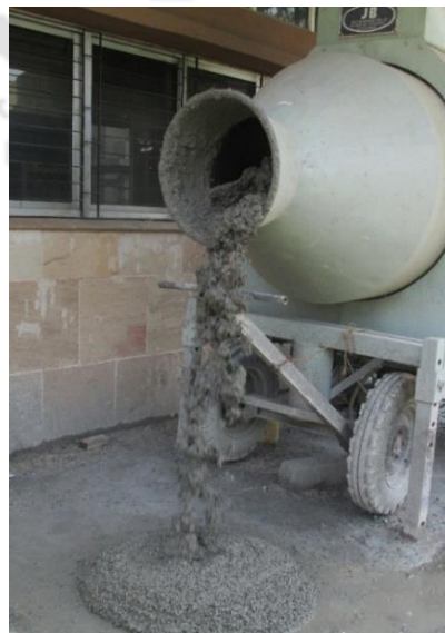
Figure 5.3. Mixing of concrete in a mechanical drum type mixer
