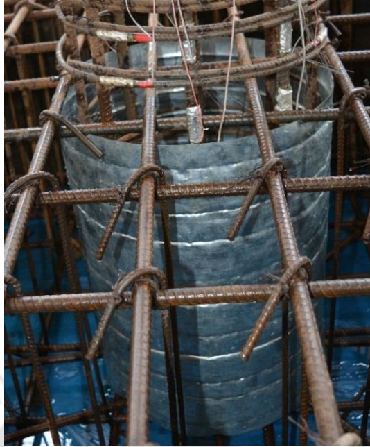
Figure 5.4. Galvanized steel tube used to separate HyFRC from conventional concrete in the footing
