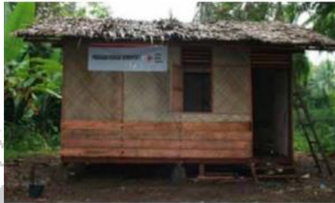
Figure 2.2: Temporary shelters build during 2009 earthquake in West Sumatra, Indonesia
