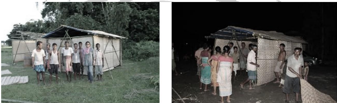
Figure 5.6 Building of Transitional Shelter with Community Participation
