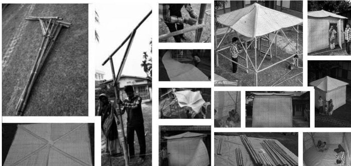
Figure 5.13. User led assembly of the Bamboo Transitional Shelter Kit
