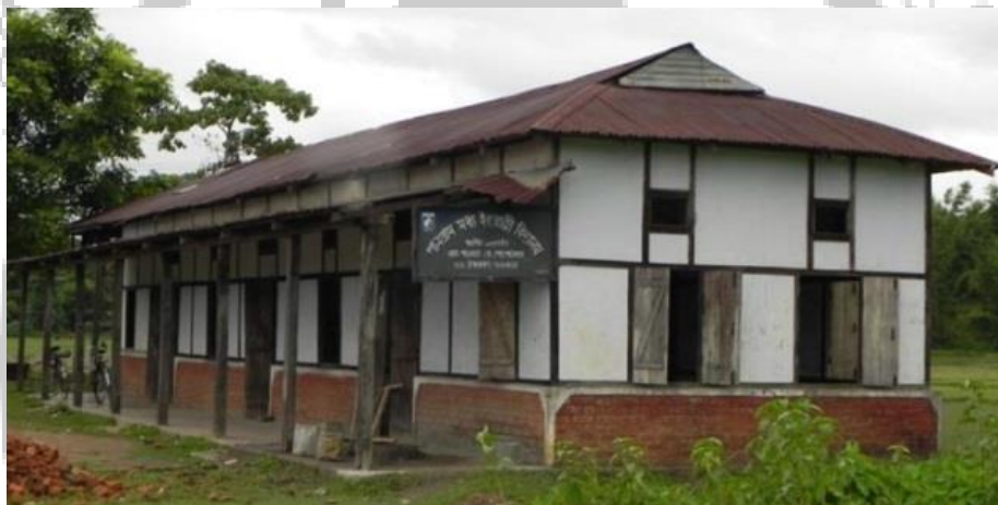
Figure4.10 View of a Typical 'Assam Type House'
