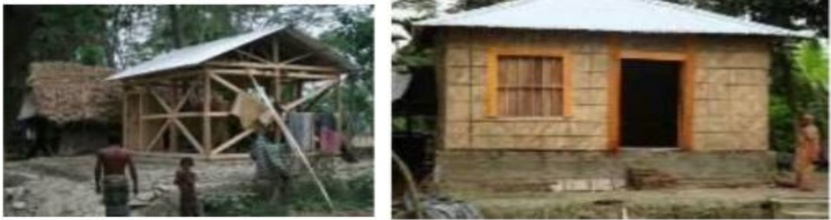
Figure 2.4: Transitional core shelter built of timber frame structure with bamboo mat walls, CGI sheet roof and earthen/bricked plinth.
