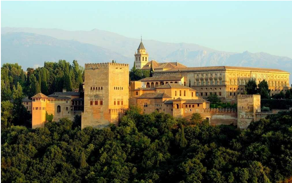
Fig. 2.7. Alhambra Fortress of Granada, Spain (constructed in 889 A.D.) (Source: Alhambra).
