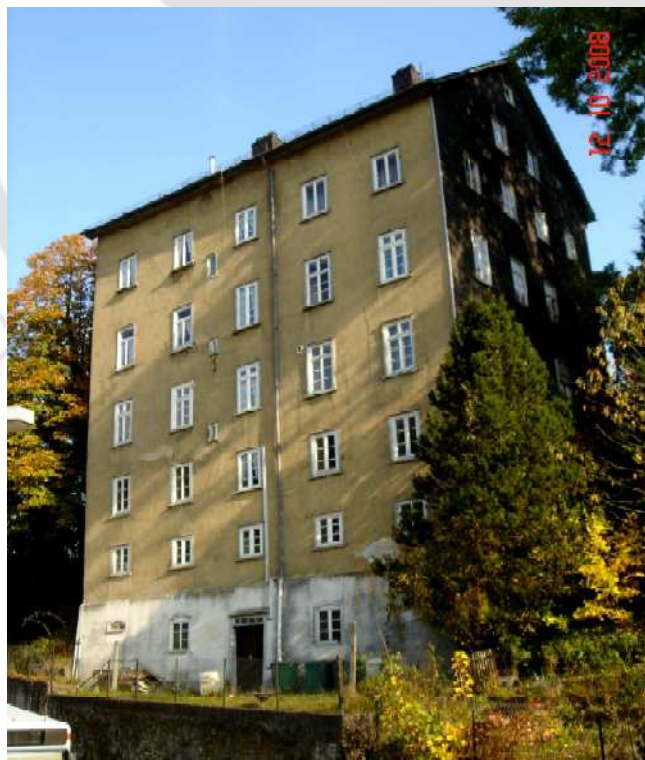
Fig. 2.8. Unstabilised rammed earth building in Weilburg, Germany (constructed in 1826 A.D.) (Source: Kumar, 2009).
