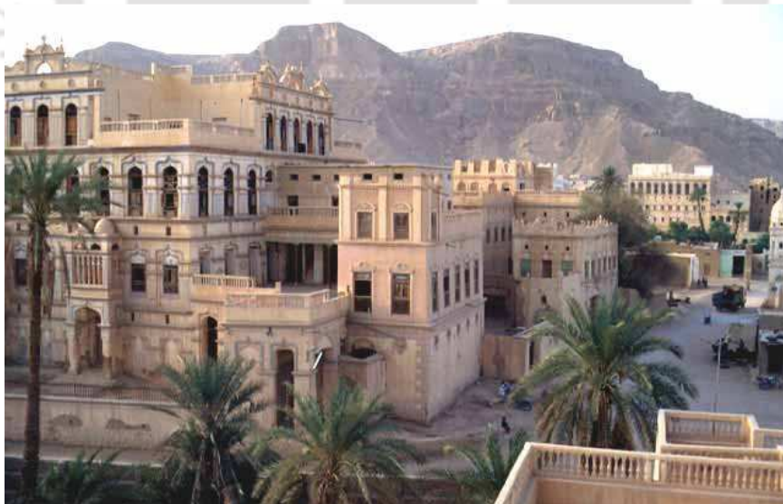
Fig. 2.6. Mud clay ancient palace in Tarim city, Yemen (constructed ~300 years ago) (Source: Helfritz, 1937).
