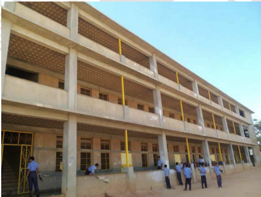
Fig. 2.12. Rammed earth school building in Bangalore, India ( Source: Reddy et al., 2014).
