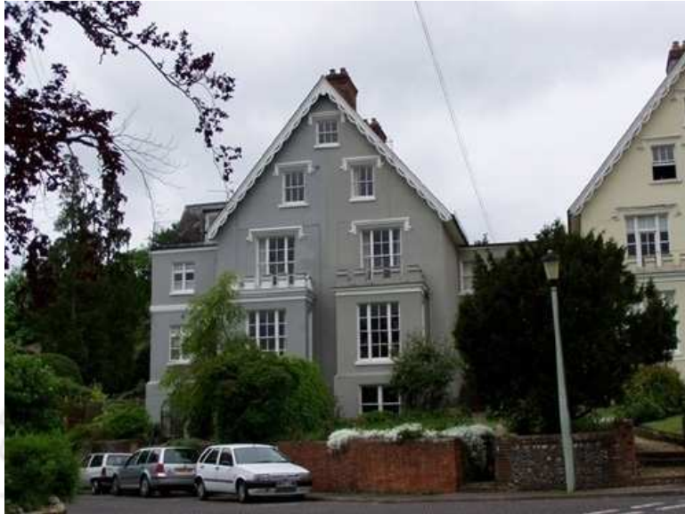
Fig. 2.9. Rammed earth chalk building in Winchester, Hampshire, UK ( Source: Kumar, 2009).
