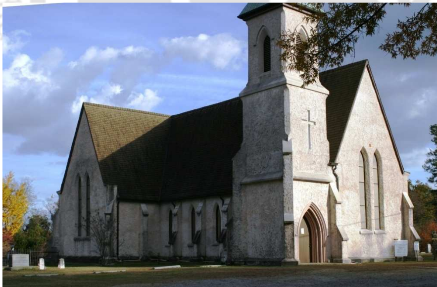
Fig. 2.10. The Church of the Holy Cross in Stateburg, South Carolina, USA (constructed in 1857 A.D.) ( Source: Wikipedia).
