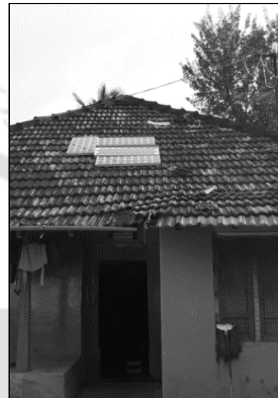
Figure 2.6 Rooftop solar panel off-grid
