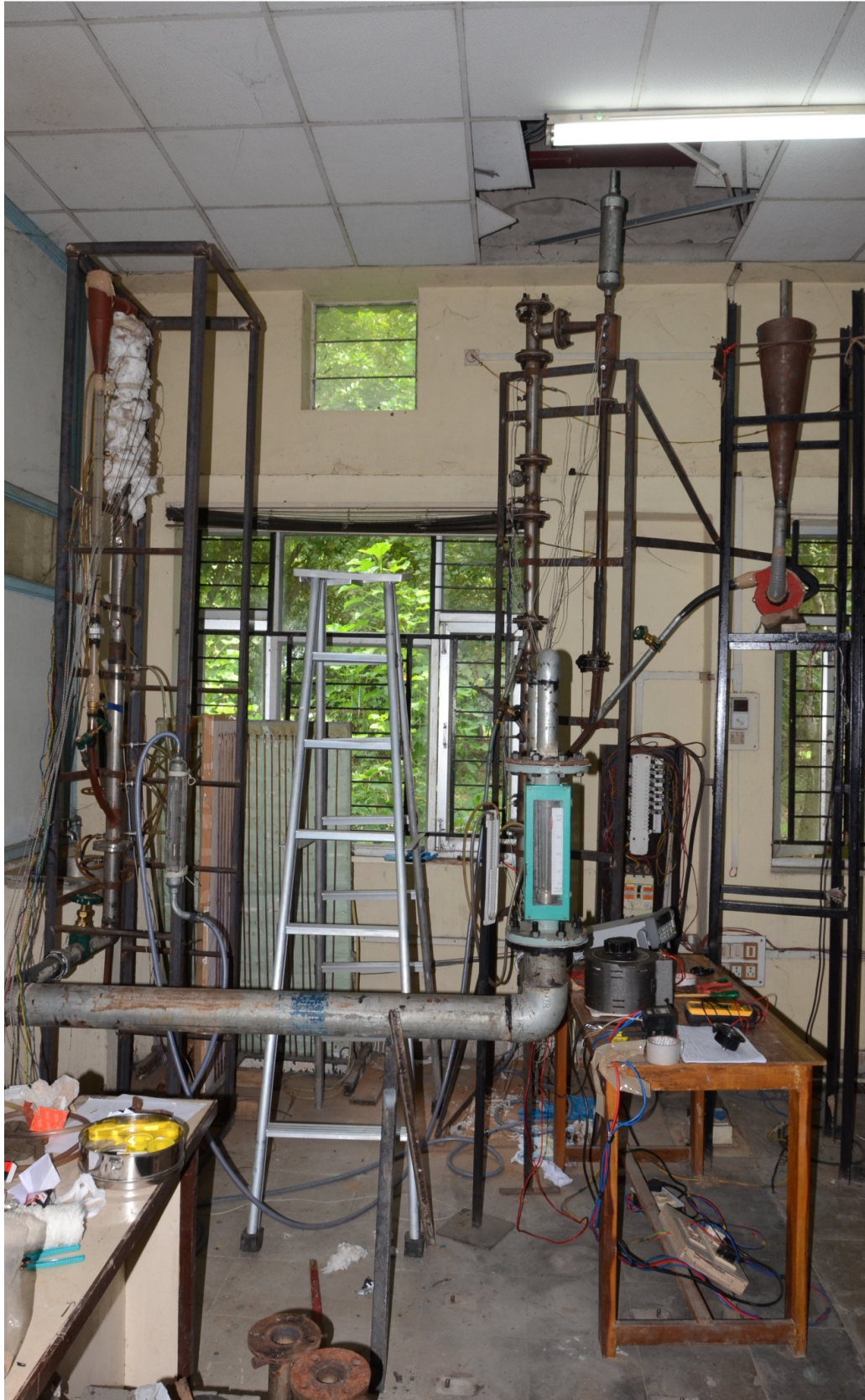
Fig.3.8 Photograph of cold and hot PCFB units
