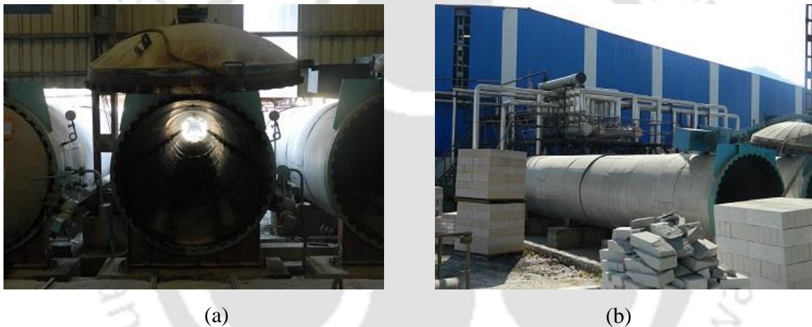
Figure 1.7 Photographs of hydrothermal treatment of green cake: (a) autoclave chamber and (b) final AAC block after autoclaving
