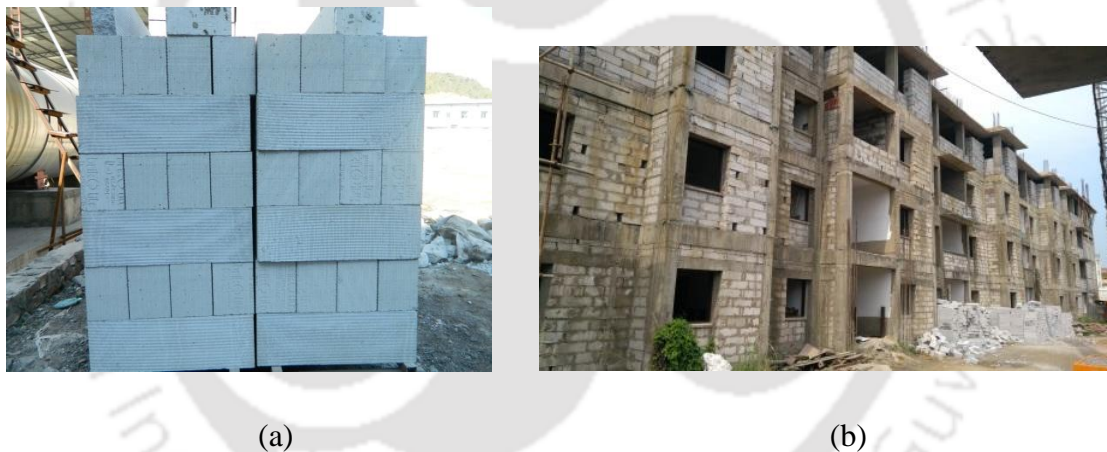
Figure 1.1 Photographs of AAC block (a) stack of AAC block and (b) building infill wall made of AAC block (Dishang Boys' Hostel, IIT Guwahati, Assam, India)
