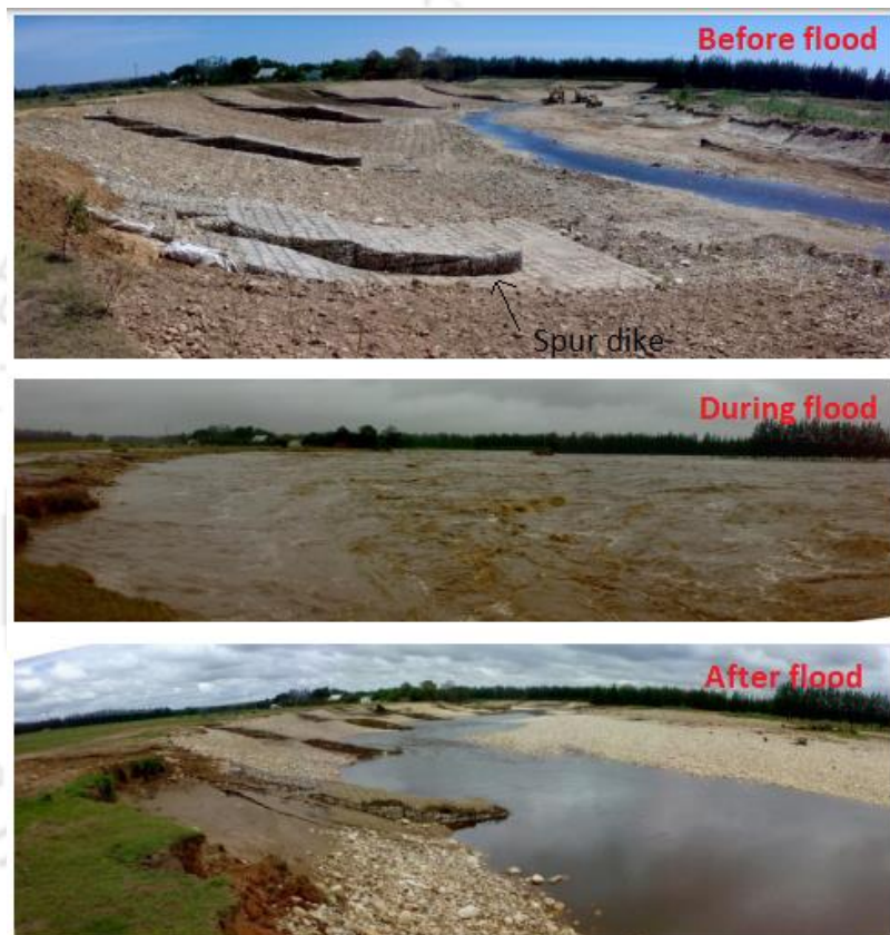
Figure 1.2 Photos captured downstream of the spur dike before, during, and after the floods in 2008, showing the minimal damage caused by the flood (King, 2009).
