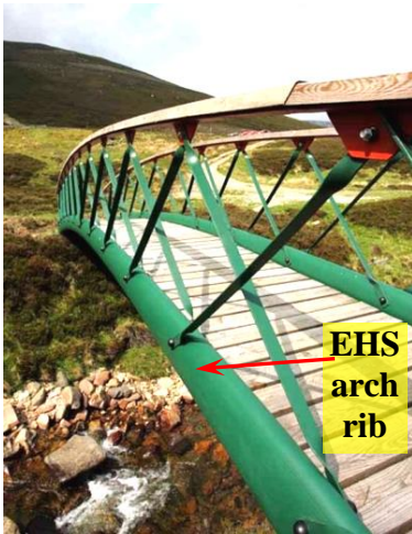
a) Highland Society Bridge, Braemar, UK [Source: Chan et al. (2010b)]
