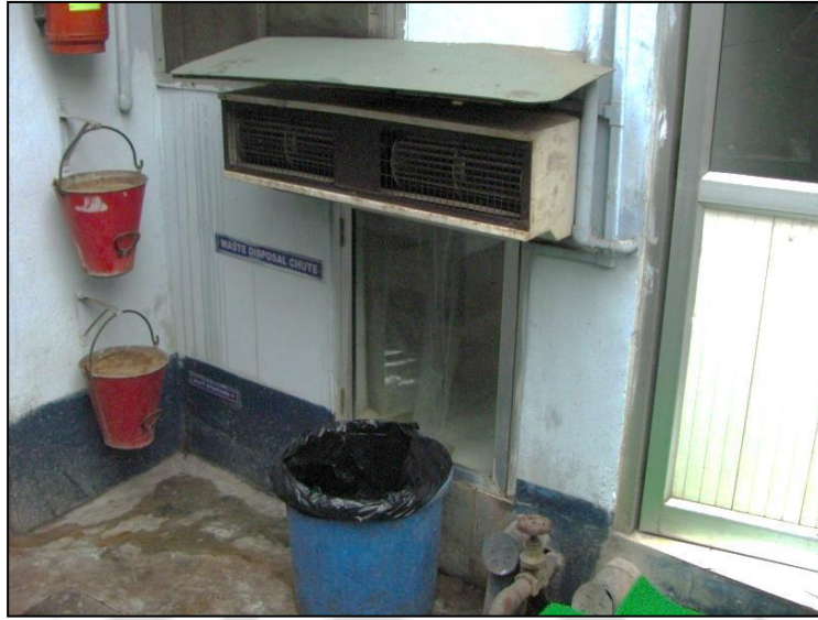
Figure 14: Waste collecting chutes at the Base kitchen Guwahati
