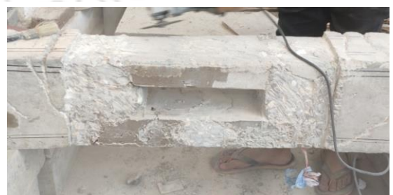
j) Repaired beam before wrapping wire mesh
