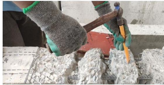
f) Chipping of concrete using chisel
