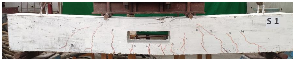
b) Crack pattern in BMS
