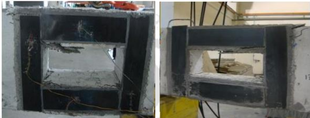
Figure 1.10: Externally bonded a) CFRP plates and b) Steel plates (Ahmed et al., 2015)
