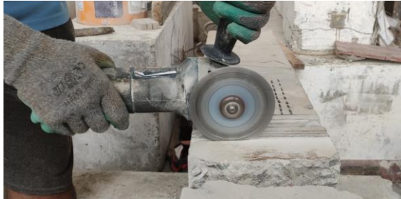
c) Cutting of concrete with grinder
