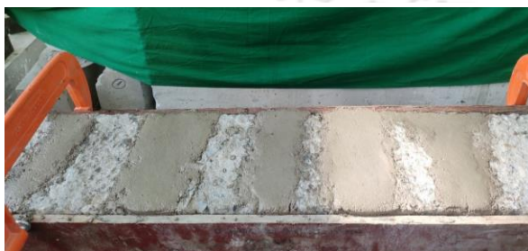
i) Filled cracks with mortar
