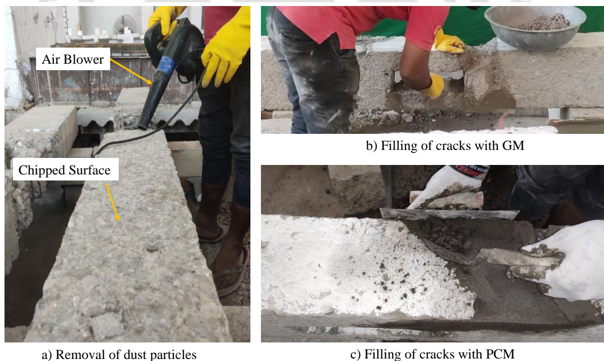
Figure 6.3: Repairing process of damaged beam
