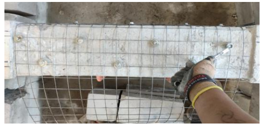
b) Fitting of wire mesh
