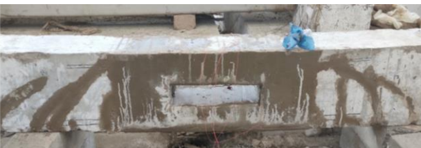
h) Repaired beam with opening in Flexural zone
