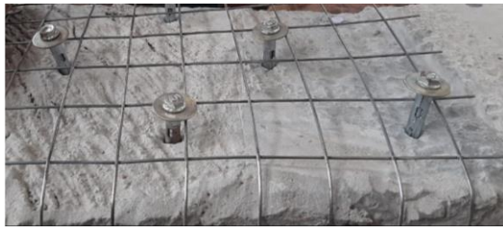
a) Installing of drop bolt anchor
