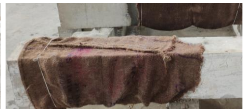
i) Curing of repaired beam
