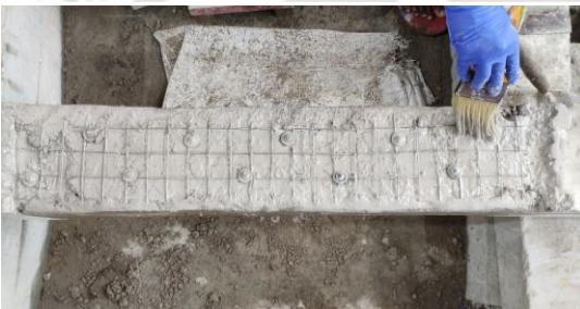
d) Application of GP for bonding
