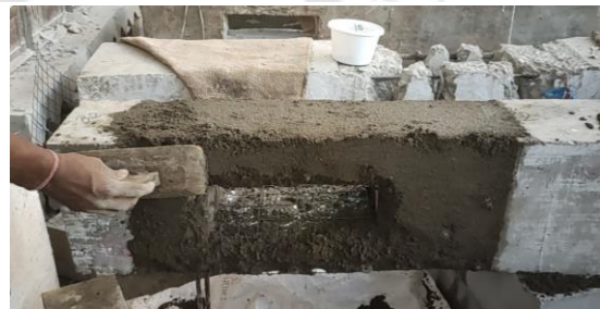
e) Application of PCM over wire mesh
