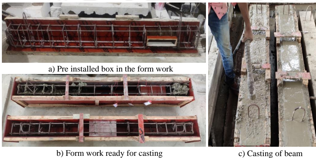
Figure 5.4: Preparation of Beam specimen
