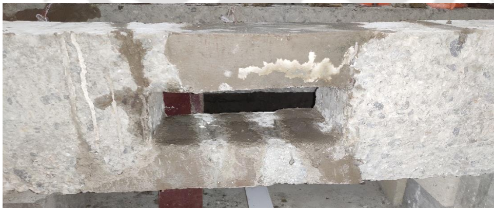
Figure 6.4: Repaired beam with opening in the flexure zone
