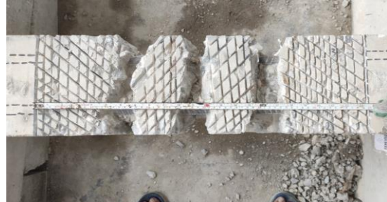
d) Surface preparation (Bottom chord)
