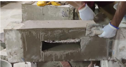
f) Finishing of GM over wire mesh
