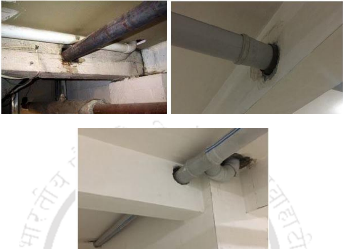
Figure 1.7: Transverse Opening in beams, Jabbar et al. (2016) and Ozkılıç et al. (2022)
