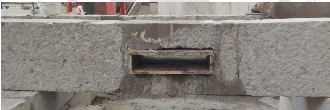
Figure 6.7: Pre-installed wooden box
