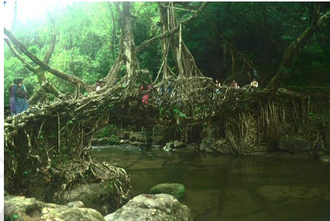
Figure 19. Living Roots bridge in Meghalaya (India).
