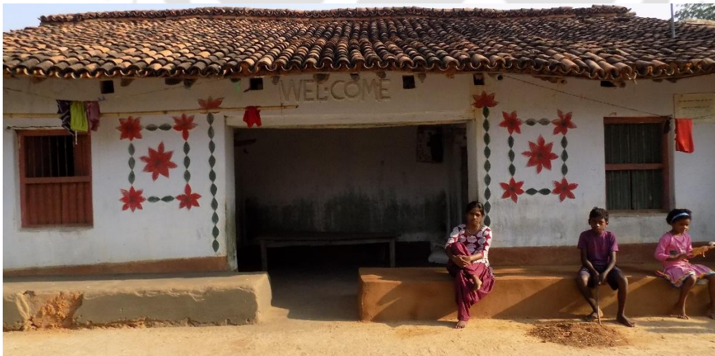
Fig. 114 Placement of visual form and use of Ota (sitting platform) and upper elevation of the wall, Dumka
