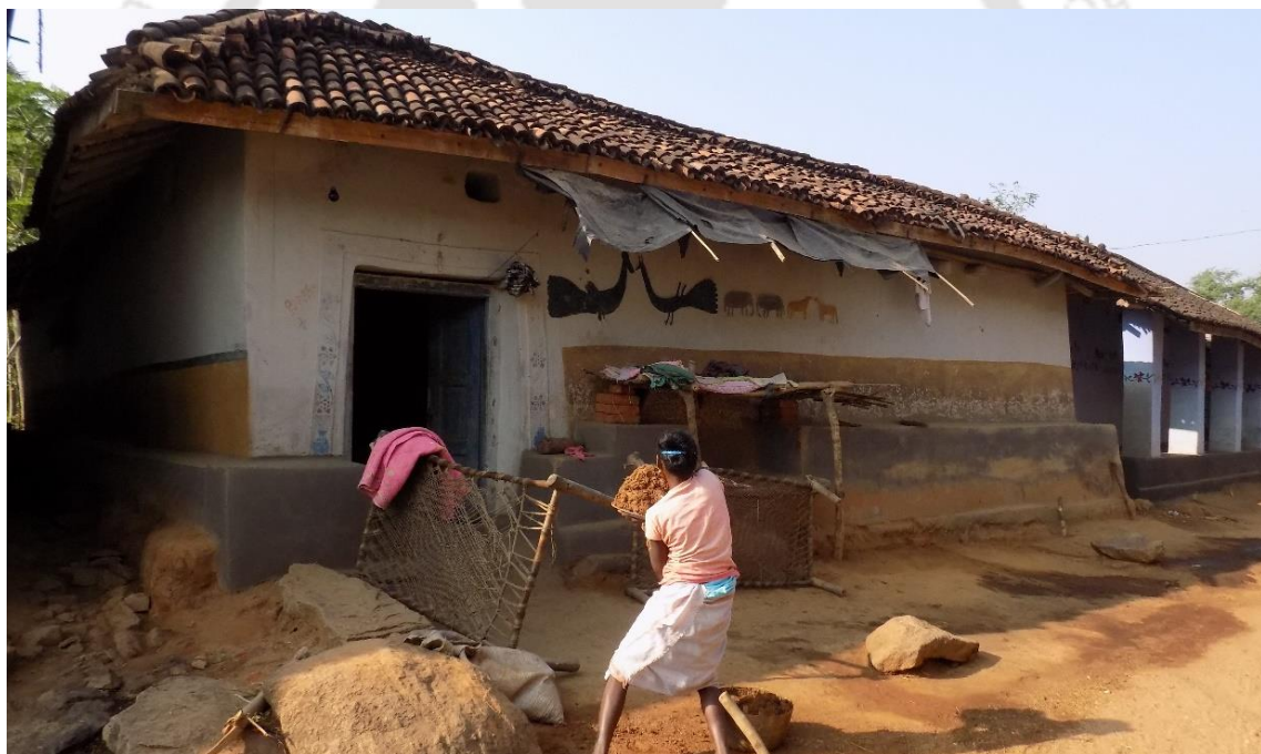
Fig. 112 Overhanging roof and space in front of the Baha bhitt (front wall)
