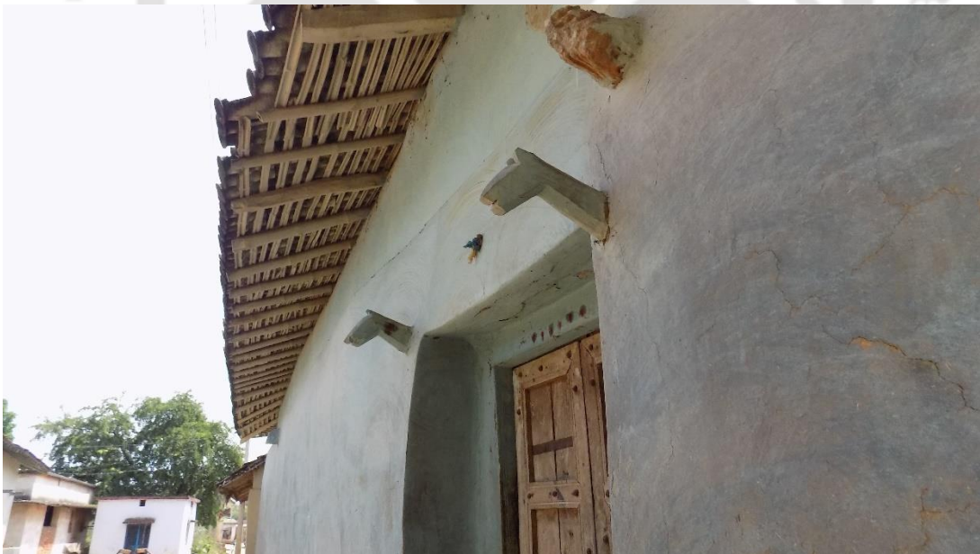
Fig. 127 Wooden horse head at the doorway
