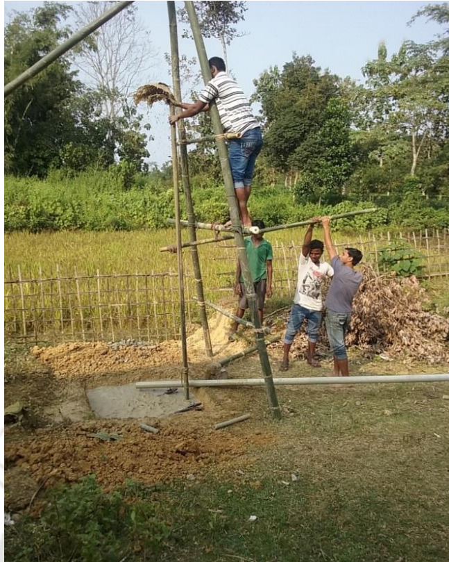
Figure 4.8 Drillers using Hand Flapping method used for drilling borewells in the study area
