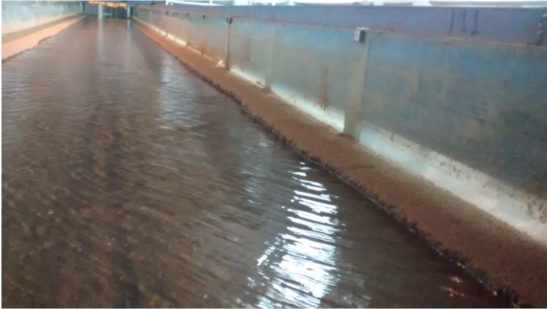
FIGURE 3.39: Distorted channel bank during the seepage experiment
