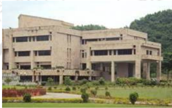
Fig. 7.10 Photograph of the torsionally coupled building
